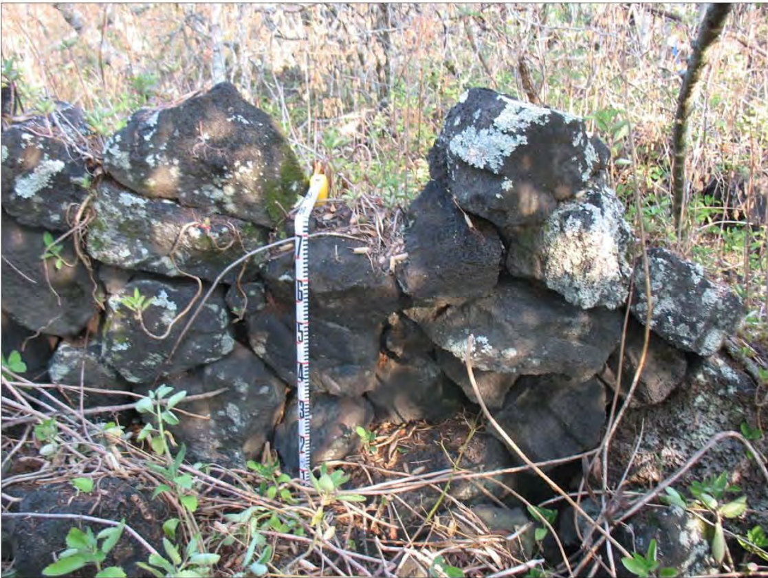
Figure 77. Site 26909, Site 488 Wall, view to north
