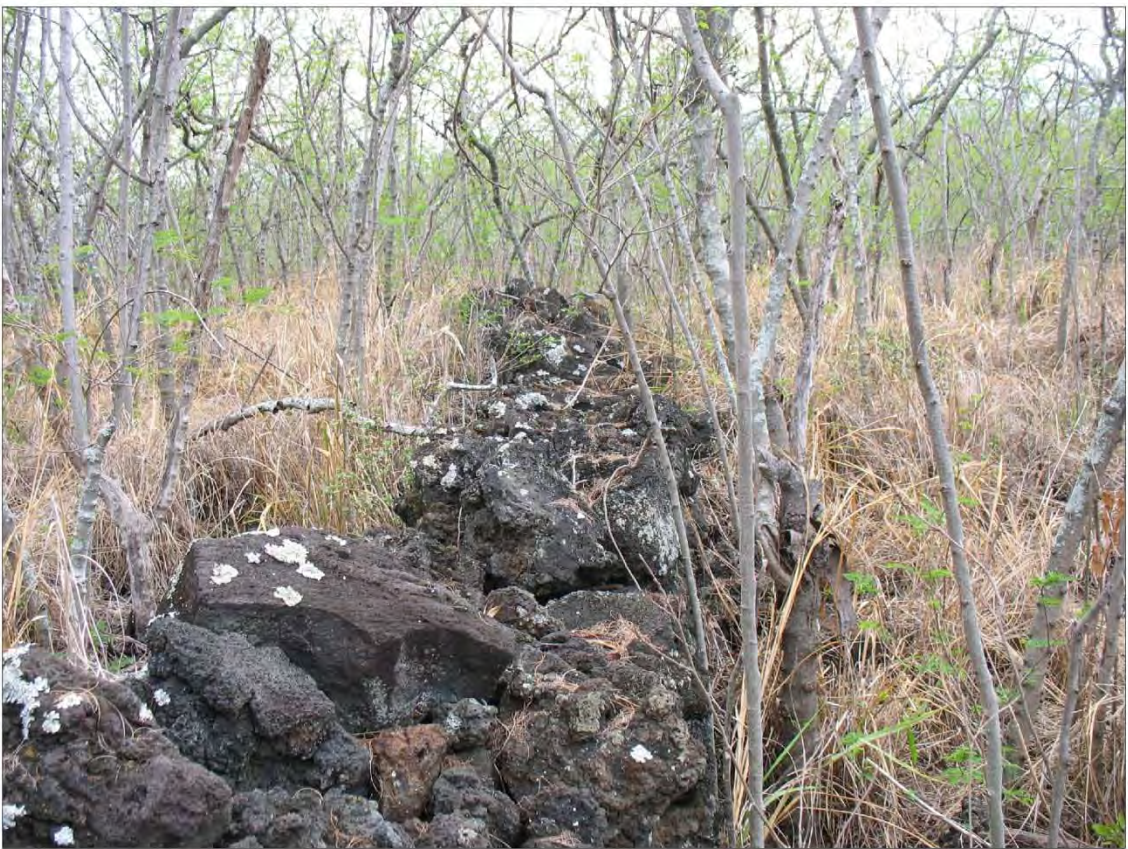
Figure 183. Site 28456, Feature A, Enclosure Wall, view to northeast
