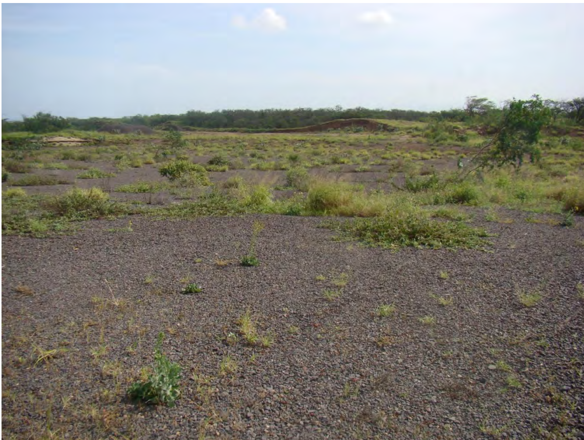
Sampling Area 3 - Sand excavation site, leveled and surfaced with a thin layer of gravel Partially re-vegetated with upland and facultative upland plant species.
