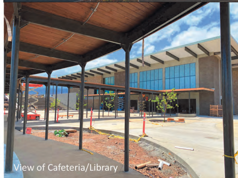
Photo Credit: Nordic PCL Construction
