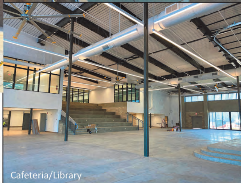
Photo Credit: Nordic PCL Construction
