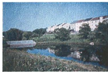
Storm water pond
