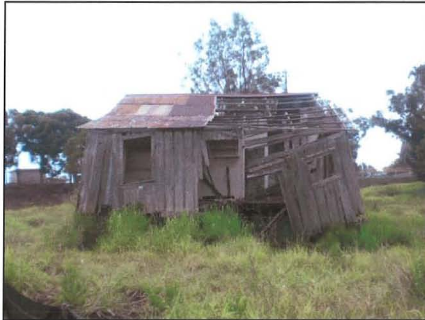
Figure 31. CSH-3, back of structure, view to north.
