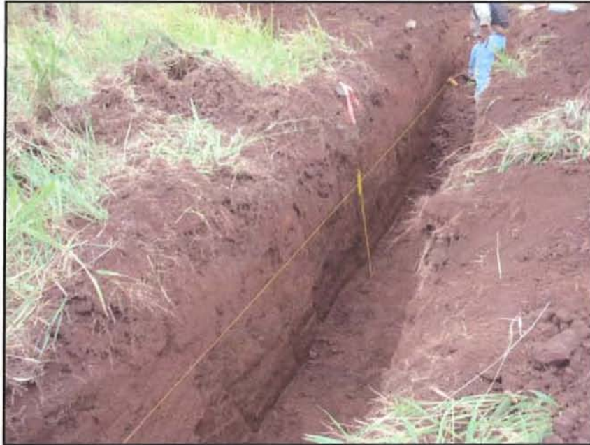
Figure 44. BT-5, 1.5m scale view to northwest
