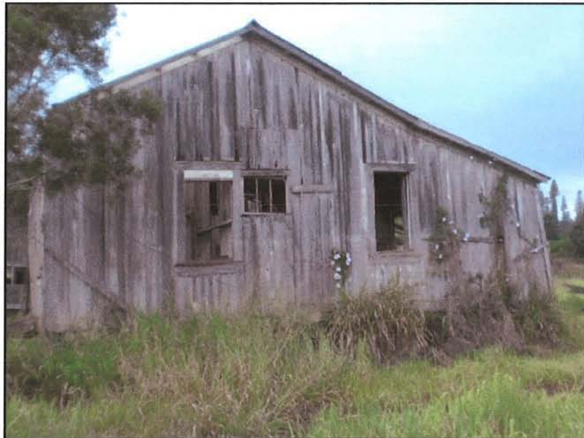
Figure 30. CSH-3, west facing wall, view to east.
