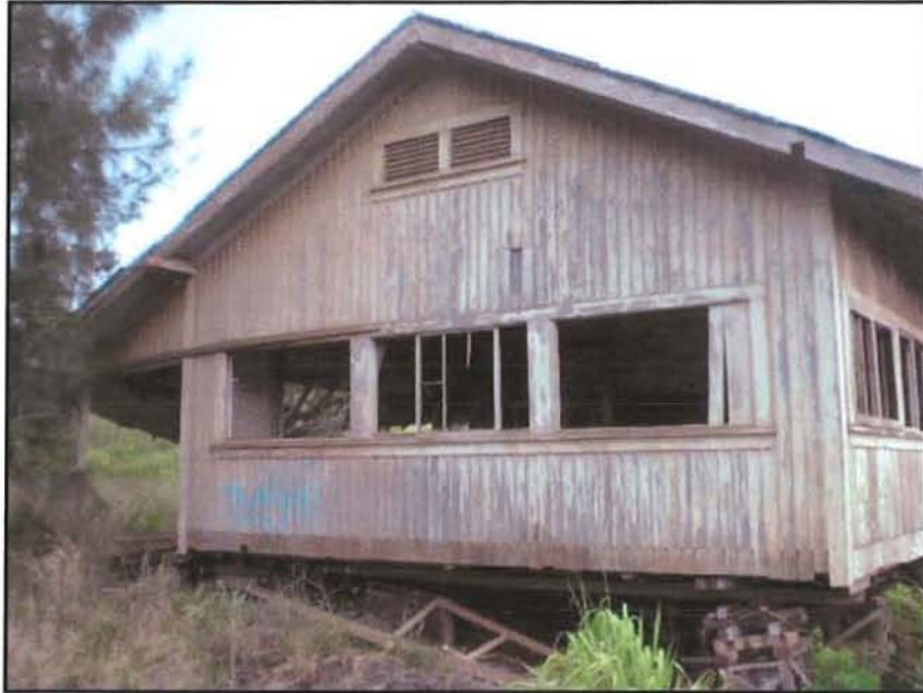
Figure 26. CSH-2, east facing wall, view to west.
