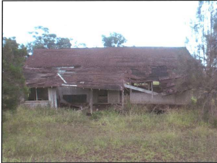
Figure 24. CSH-2, front of structure, view to north.
