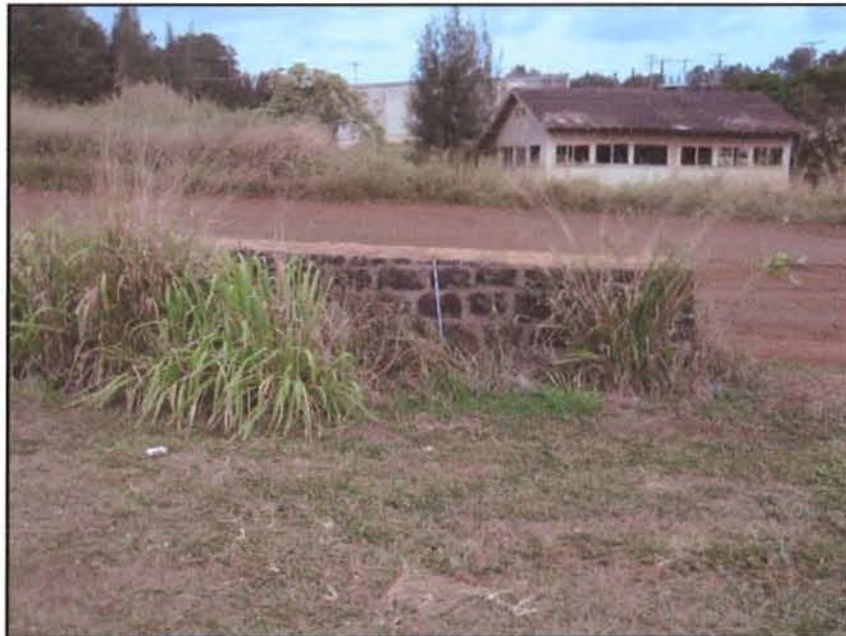
Figure 21. SIHP 50-40-98-6649, view to south.
