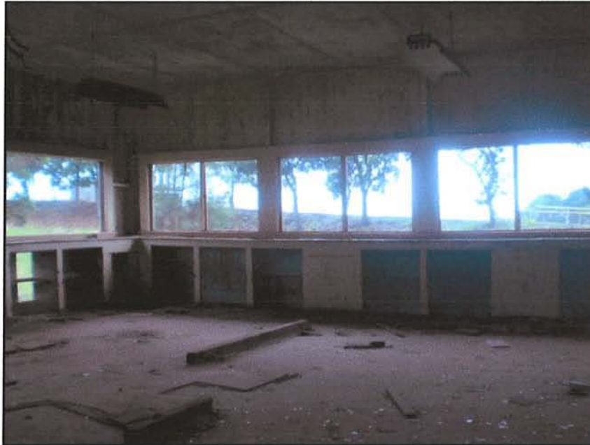
Figure 28. CSH-2, interior of room two, view to north.
