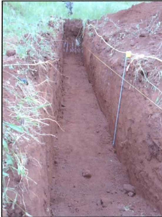
Figure 35. Overall view of BT-3, view to east.
