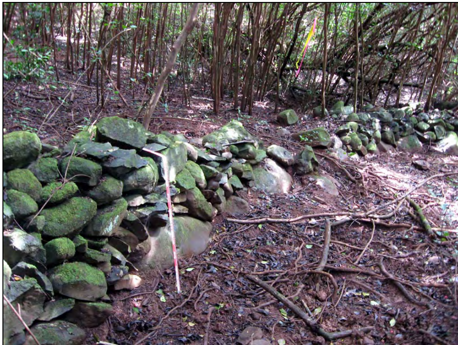
Figure 52. Photograph of SIHP # 50-80-09-7044 N stream channel improvements, showing stacked-stone wall, view to south
