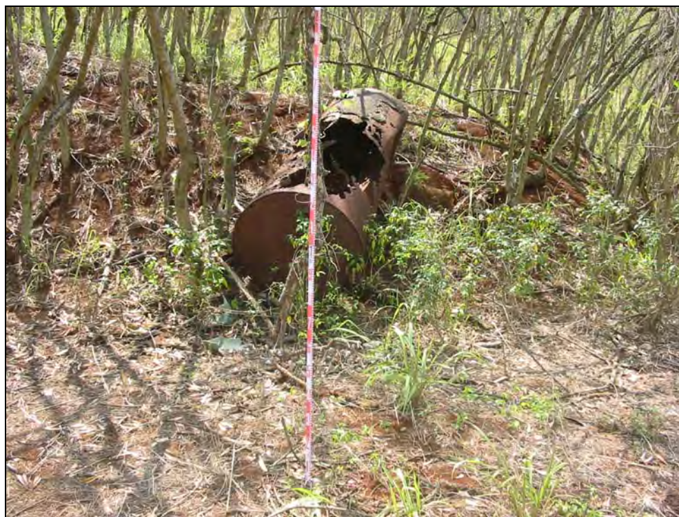
Figure 99. Photograph of SIHP # 50-80-09-7052 C concrete building foundation, showing metal tank, view to southeast
