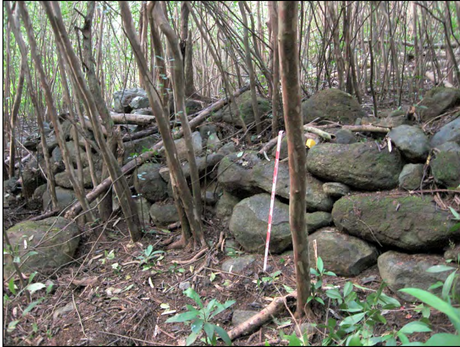
Figure 57. Photograph of SIHP # 50-80-09-7044 Q stream channel improvements, showing retaining wall, view to north
