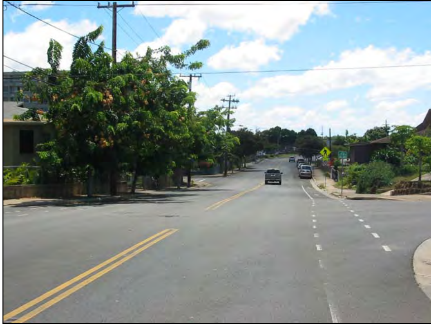
Figure 34. Photograph of asphalt paved streets within makai project area, taken at Mokuloa Street, view to southeast
