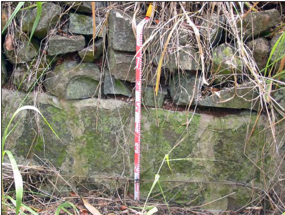
Figure 106. Photograph of SIHP# 50-80-09-9530 A irrigation ditch, showing cut basalt block lining with stacked basalt cobbles above, view to east
