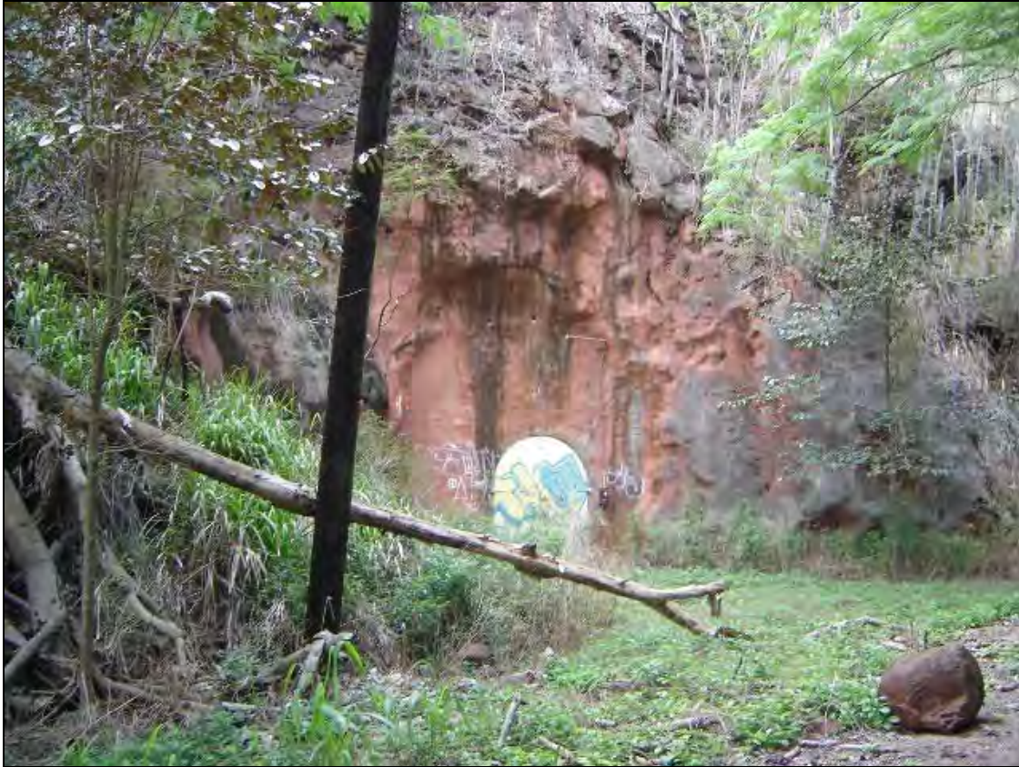
Figure 20. Mr. Kalahiki participated in the construction of this military bunker in Kīpapa Gulch
