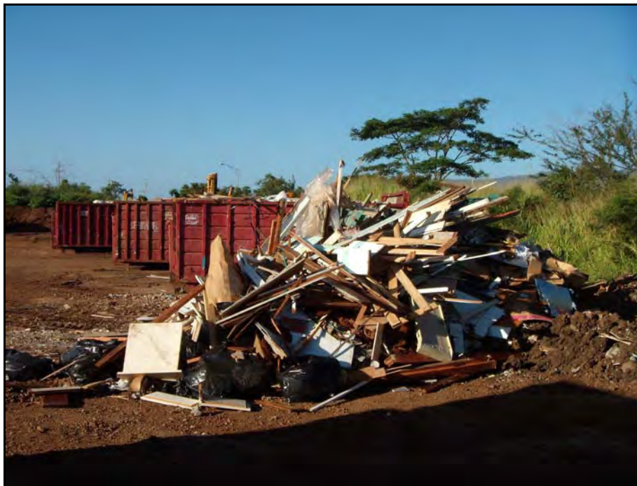
Figure 10. Portion of the Department of Transportation staging area showing degree of disturbance facing west
