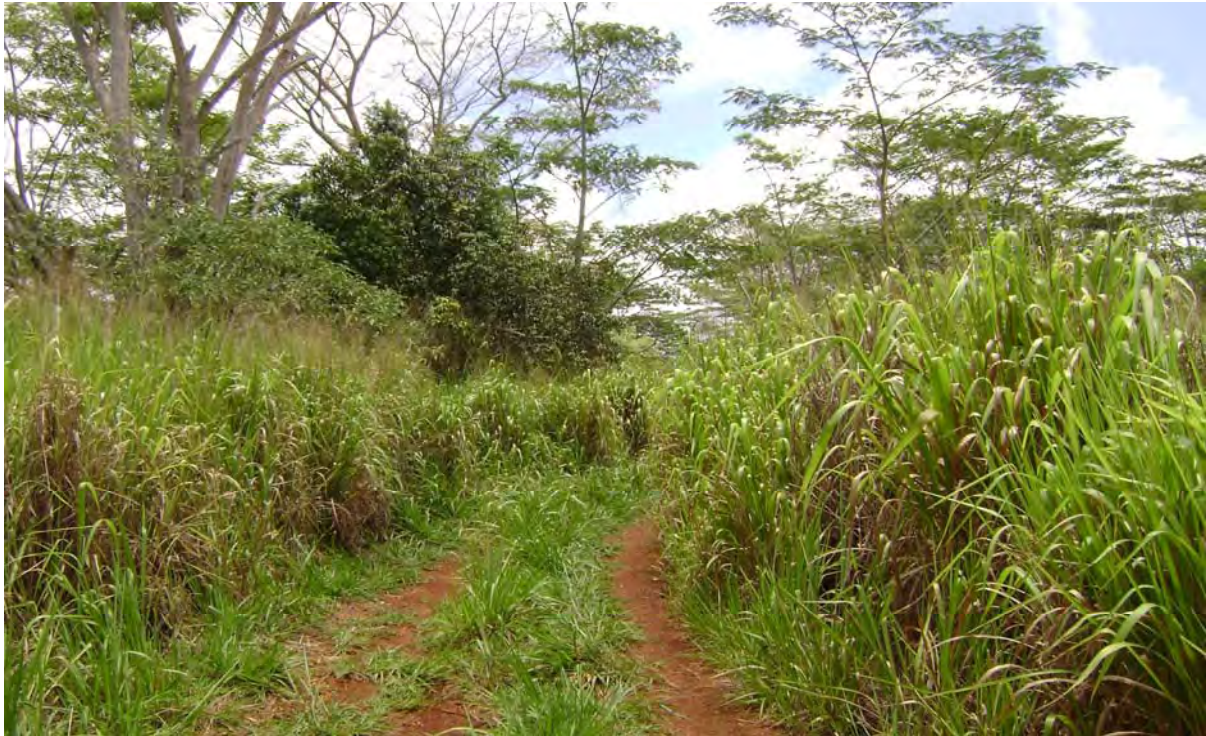
Fig. 6. Guinea grass overgrowing infrequently used unpaved road.
