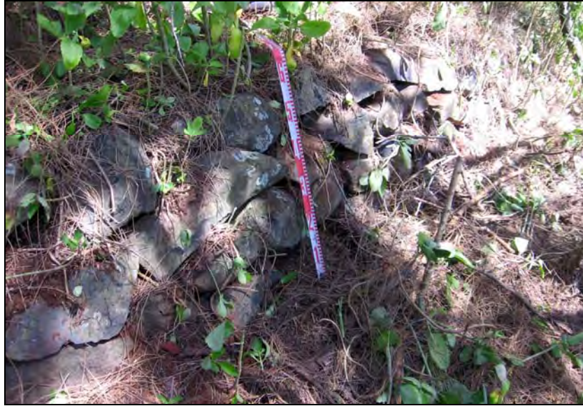
Figure 94. Photograph of SIHP # 50-80-09-7051 retaining wall, view to northwest
