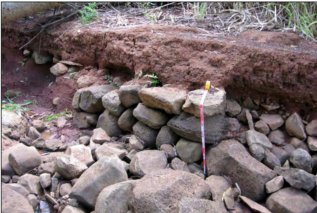
Figure 90. Photograph of SIHP # 50-80-09-7049 J retaining wall, view to southwest
