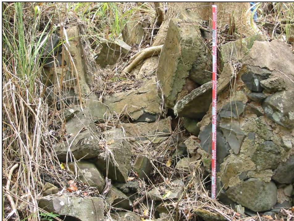
Figure 121. Photograph of SIHP # 50-80-09-9530 E irrigation ditch, showing sluice gate, view to east
