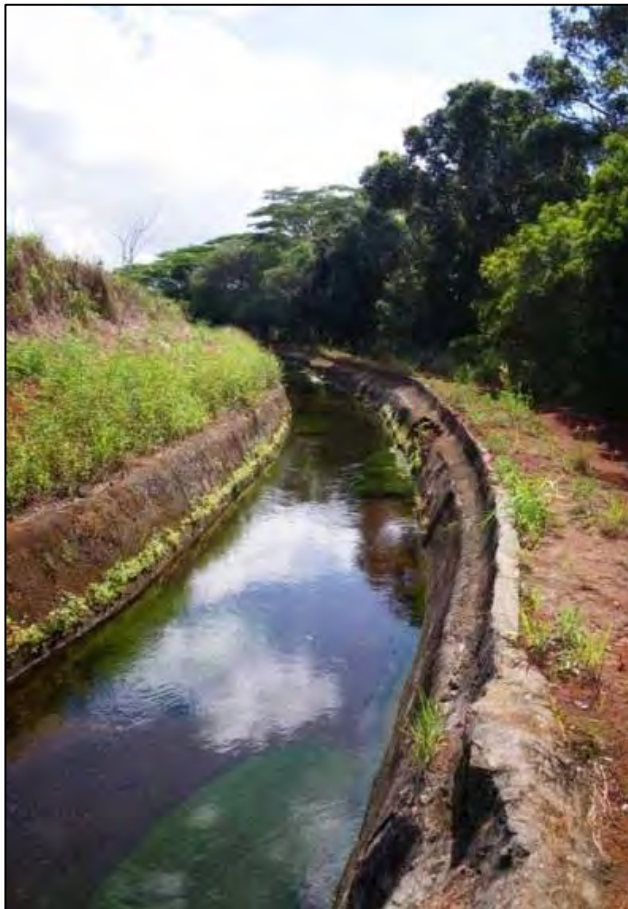
Figure 6. Section of Waiāhole Ditch as it passes through the property.
