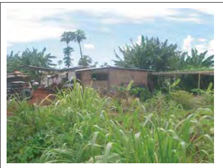
Photograph 6: Shed structure located on the south portion of the Subject Property.
