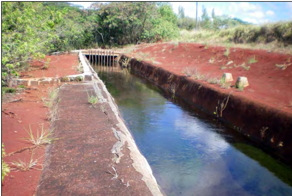
Figure 33. Photograph of SIHP # 50-80-09-2268 Waiahole Ditch, showing open ditch and siphon entrance, view to northwest
