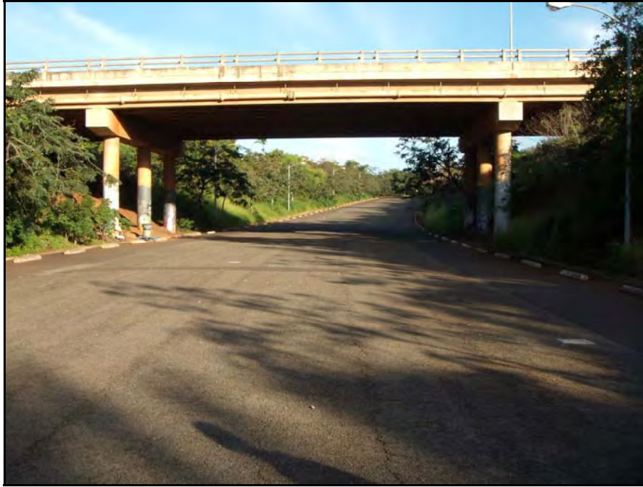
Figure 30. Photograph showing bus parking lot elevation in relation to surface streets as well as surrounding road cuts, view to northwest
