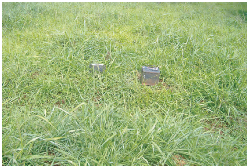
Photograph 4: Batteries located on the north portion of the Subject Property.
