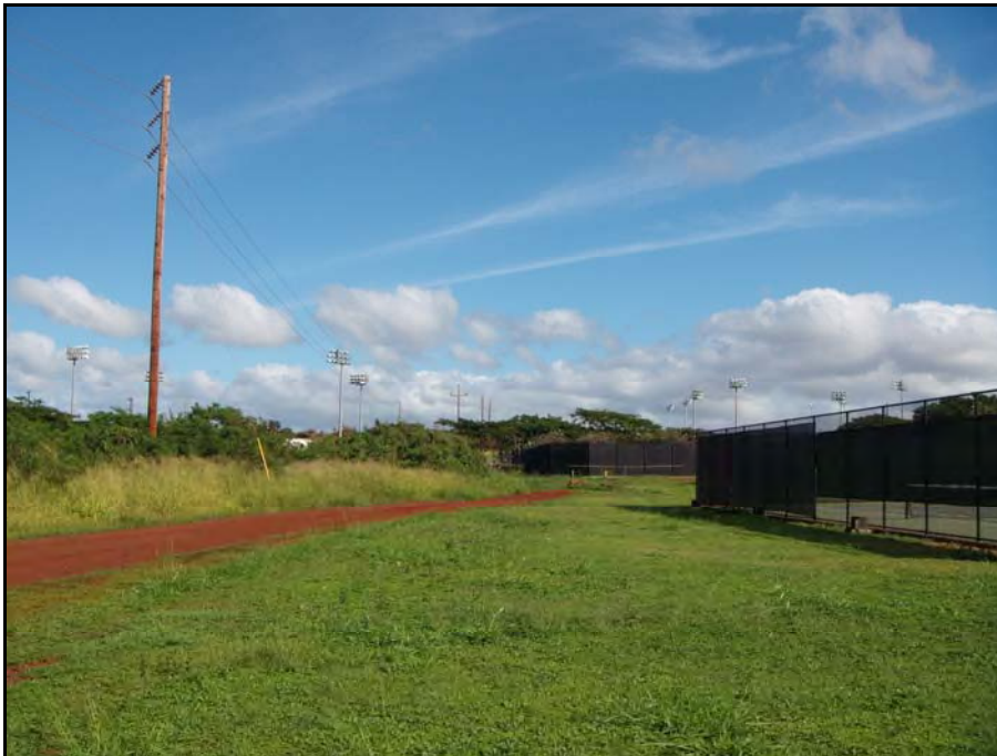
Figure 33. Photograph of the modern power line corridors and park facilities bordering the northern portion of the mauka project area, view to north
