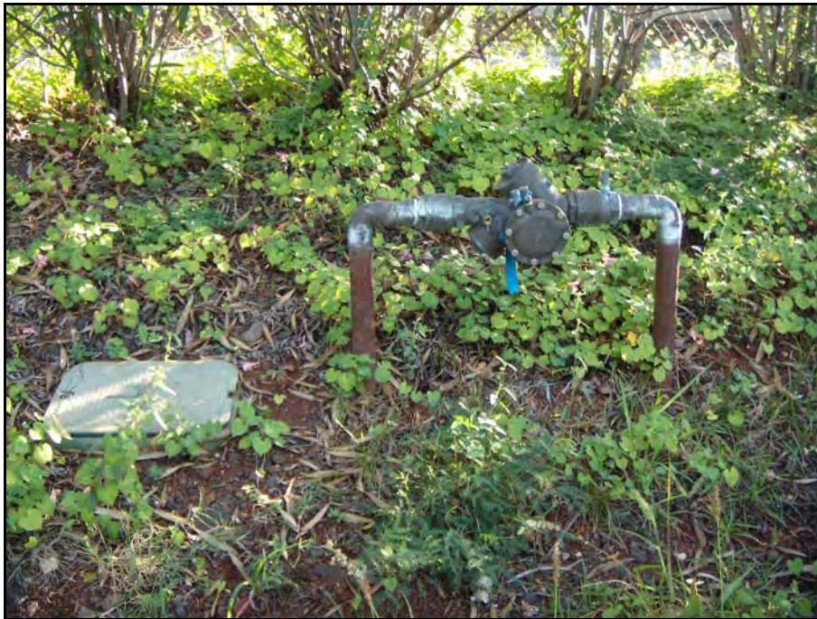
Figure 31. Photograph of modern utilities along road cut, view to northeast
