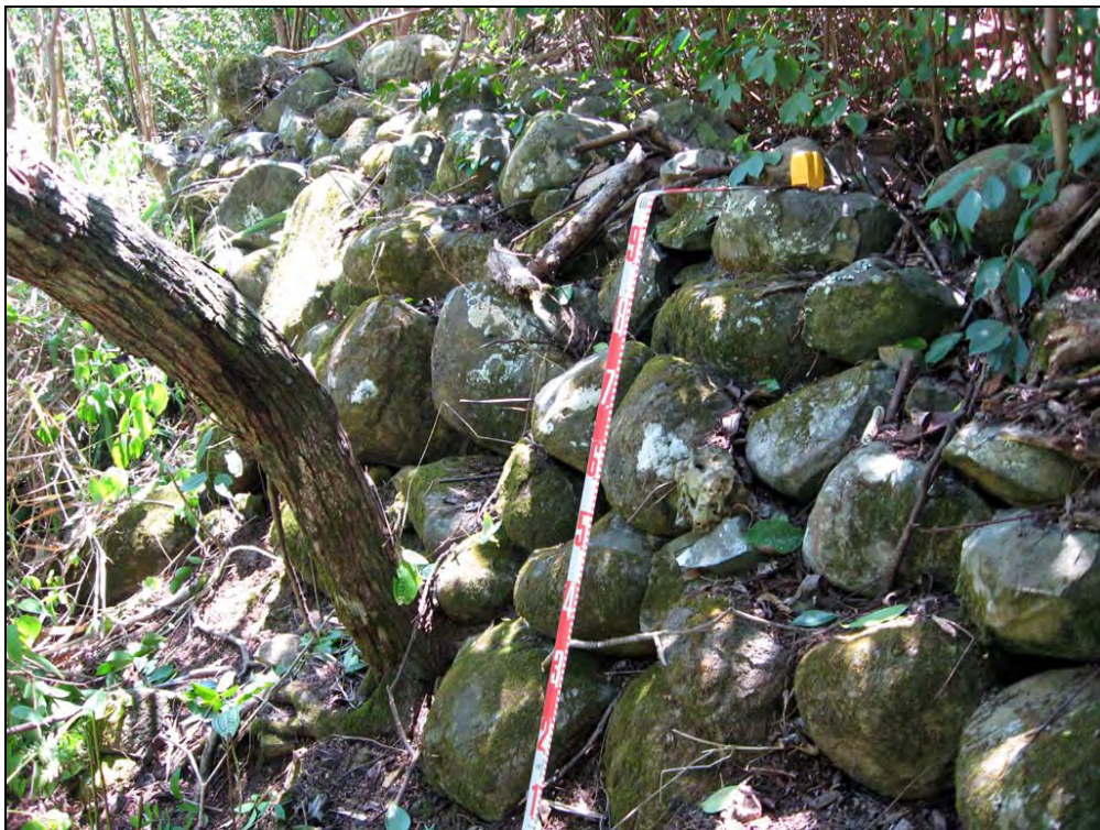
Figure 84. Photograph of SIHP # 50-80-09-7049 E terrace, view to south
