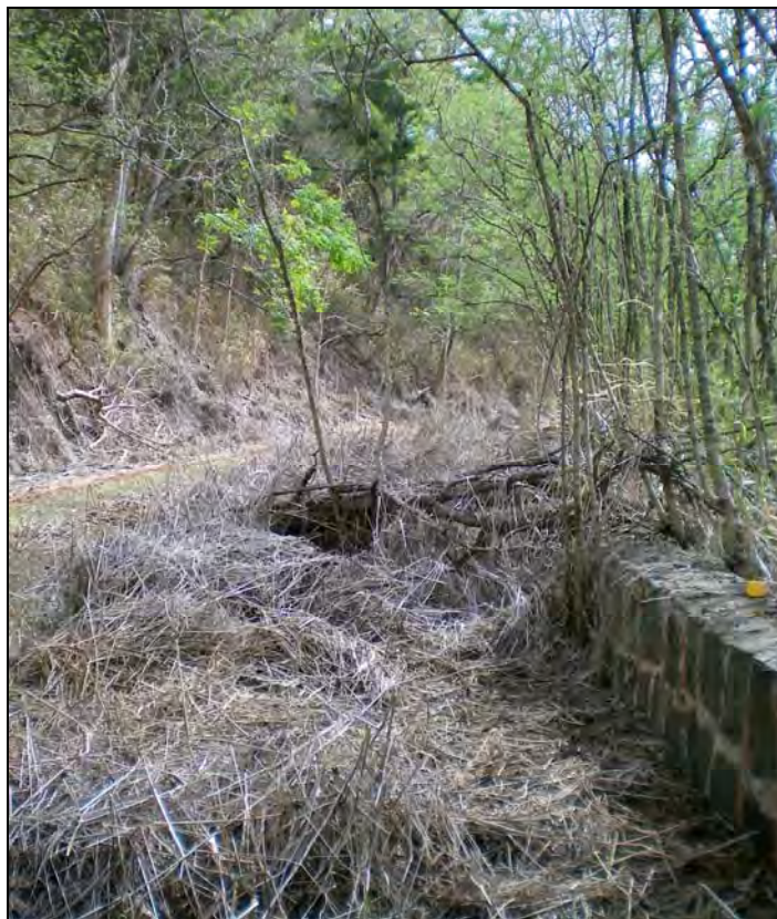
Figure 100. Photograph of SIHP # 50-80-09-7053 Old Kamehameha Highway roadbed (Feature A), showing wall (Feature B) along down slope edge (right), view to south
