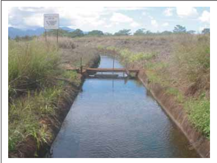
Photograph 10: Waihole Ditch located on the north portion of the Subject Property.
