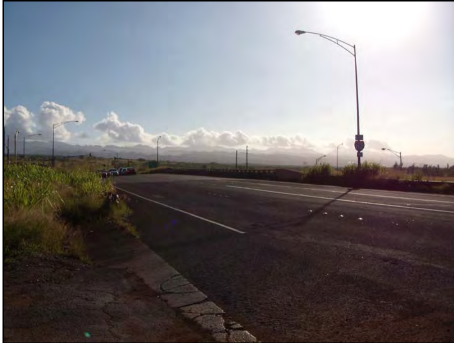
Figure 9. Ka Uka Boulevard showing I-H2 overpass facing southeast
