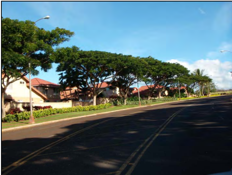
Figure 29. Photograph of a residential complex along Paiwa Street, view to northwest
