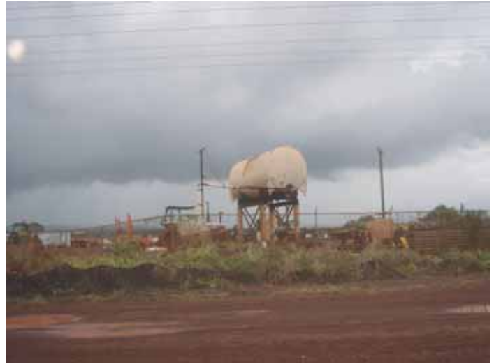
Photograph 2: Inactive fertilizer AST located within the Loading and Storage area.
