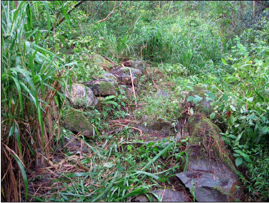
Figure 39. Photograph of northern portion of SIHP # 50-80-09-7044 C stream channel improvements, showing boulder alignment (right) and stacked-stone retaining wall (left), view to southeast
