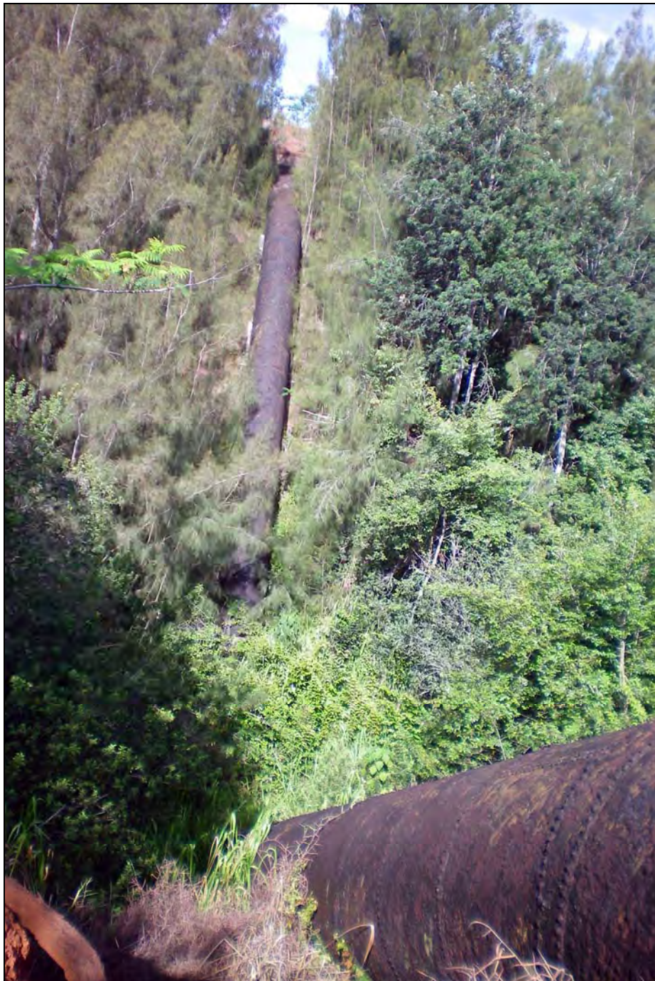
Figure 31. Photograph of SIHP # 50-80-09-2268 Waiahole Ditch, showing siphon across tributary of Pānakauahi Gulch, view to west
