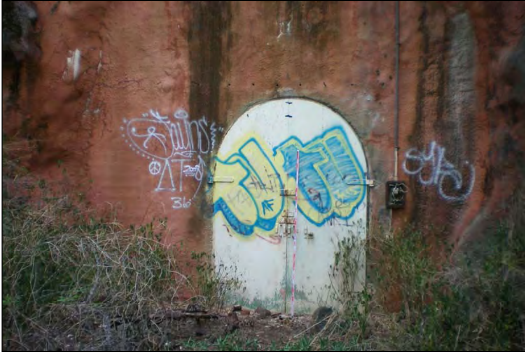
Figure 95. Photograph of SIHP# 50-80-09-7052 A ammunition storage tunnel, showing tunnel entrance, view to west
