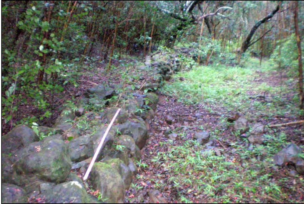
Figure 42. Photograph of SIHP # 50-80-09-7044 E stream channel improvements, showing stacked-stone wall along edge of stream channel, view to west
