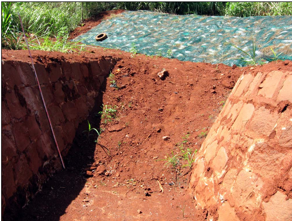
Figure 8. SIHP # 50-80-09-9530 Feature A irrigation ditch, showing earthen berm recently constructed over the ditch (views to southeast, south)
