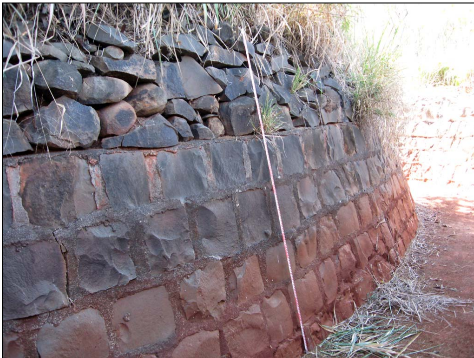
Figure 24. SIHP # 50-80-09-9530 Feature A irrigation ditch, showing additional stacked-stone lining above the cut basalt block and mortar ditch lining (view to east)
