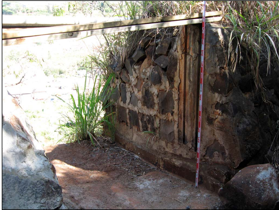
Figure 25. SIHP # 50-80-09-9530 Feature A irrigation ditch, showing sluice gate and ditch outlet at the edge of Kīpapa Gulch (view to northwest)
