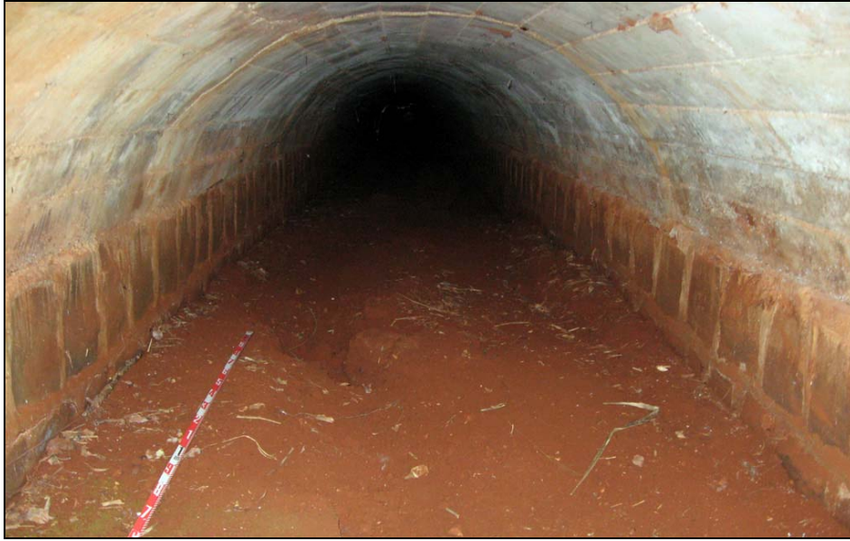
Figure 31. Photograph of the interior of the SIHP # # 50-80-09-9530 Feature A ditch tunnel
