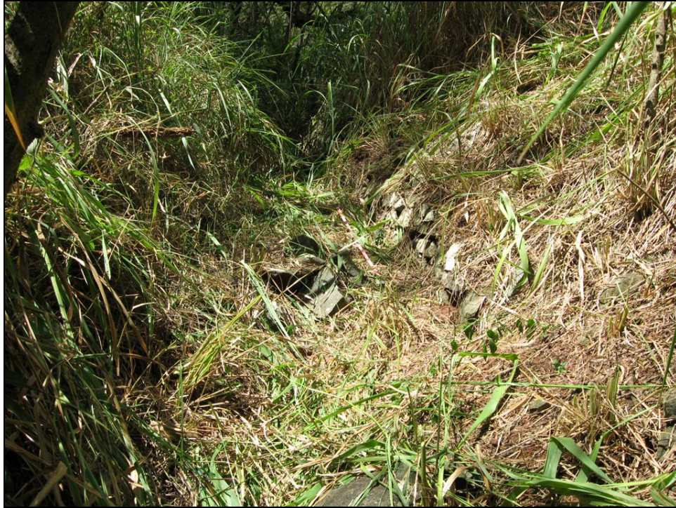
Figure 36. Photograph of SIHP # 50-80-09-9530 Feature B ditch, showing primarily earthen ditch construction with limited stacked-stone lining, view to south
