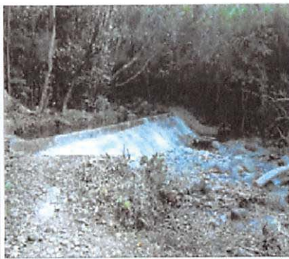
Figure 28: S. Waikapū Dam Intake Diversion (2012)
