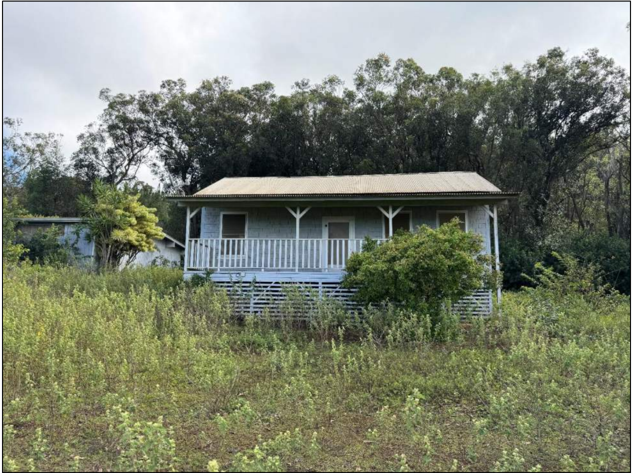
Figure 29. Front (southwest) facade of Structure C (MASON, 2024).
