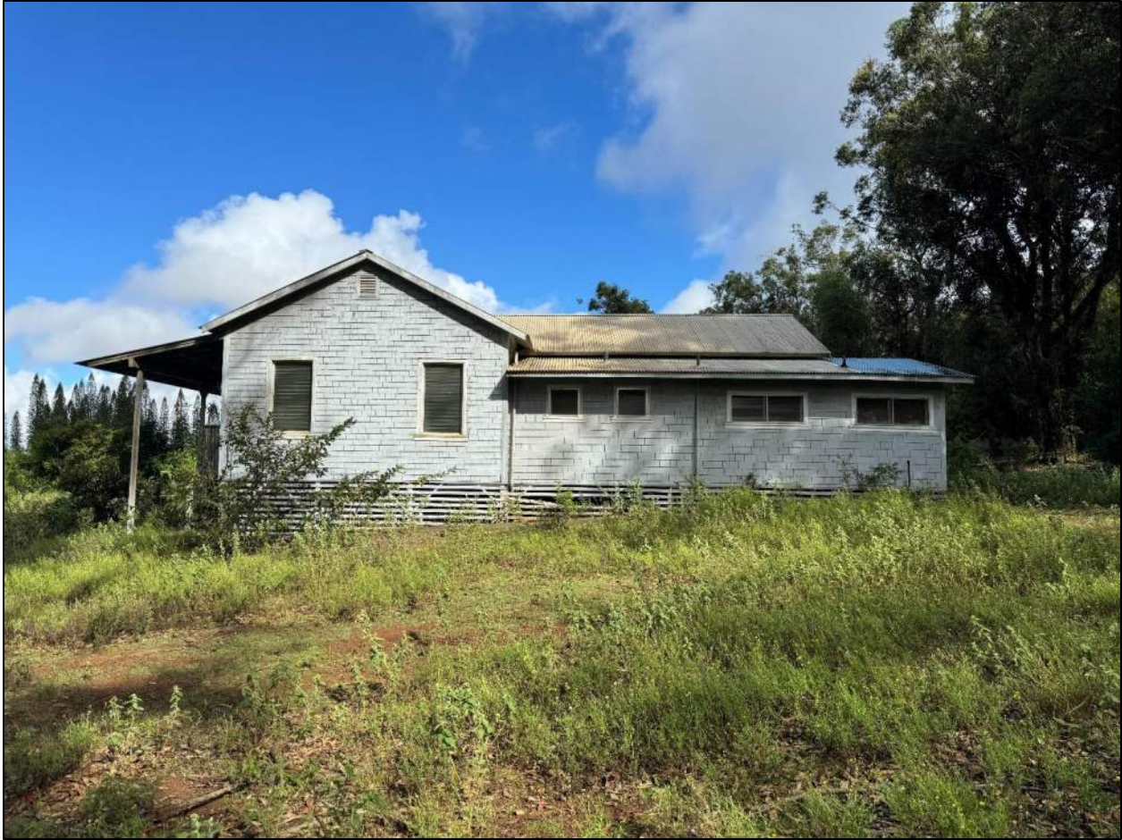
Figure 34. Structure C's southeast facade, camera facing northwest (MASON, 2024).
