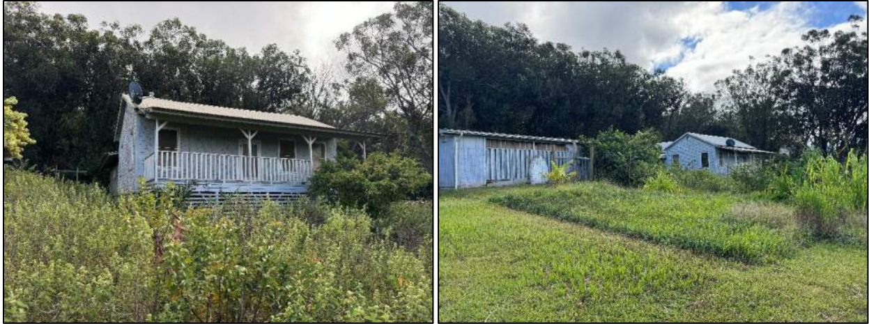
Figure 31. Structure C's southwest and northwest facades, camera facing northeast (left) and southeast (right) (MASON, 2024).
