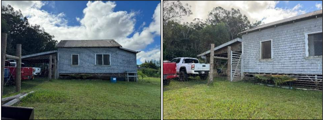
Figure 48. Structure D's northwest facade, camera facing southeast (left) and east (right) (MASON, 2024).
