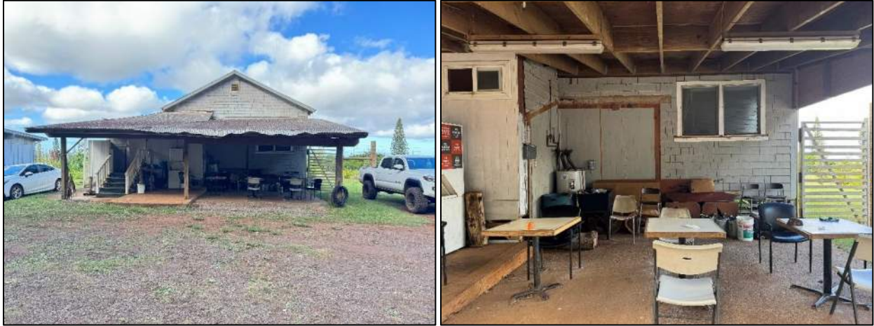
Figure 49. Structure D's northeast facade, camera facing southwest (MASON, 2024).
