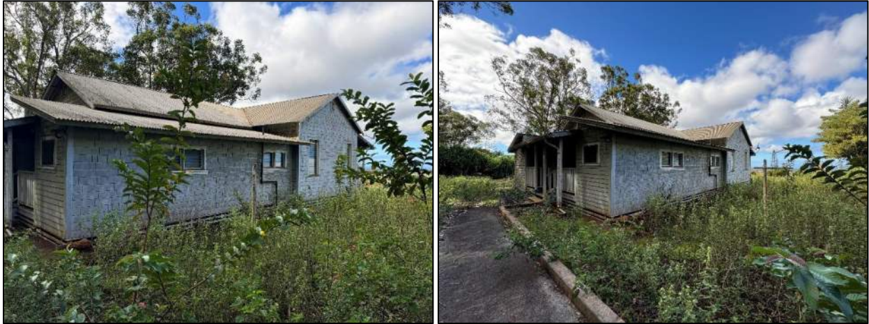
Figure 32. Structure C's northwest and northeast facades, camera facing south (MASON, 2024).
