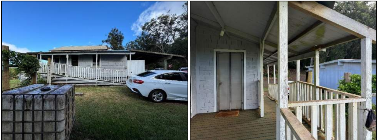
Figure 51. Structure D's southeast facade (left) and the wheelchair ramp along the southeast facade (right) (MASON, 2024).
