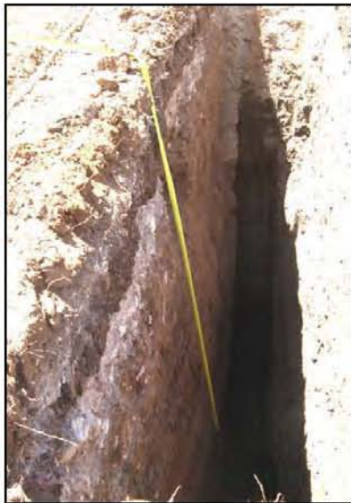
Test Trench 21, west wall showing 3.7 meters of tape ( karst bedrock not found).
