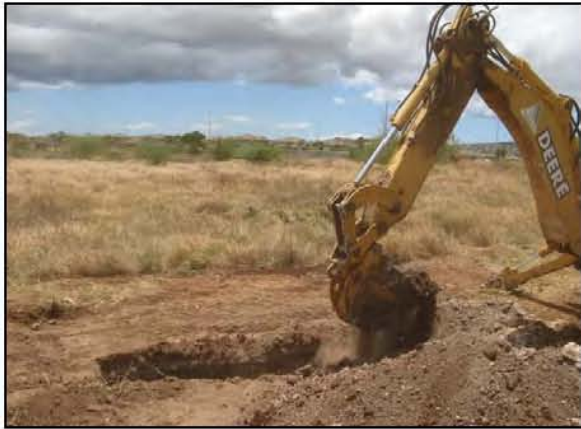
Test Trench 21 located in northwest extreme of property (view to northwest).
