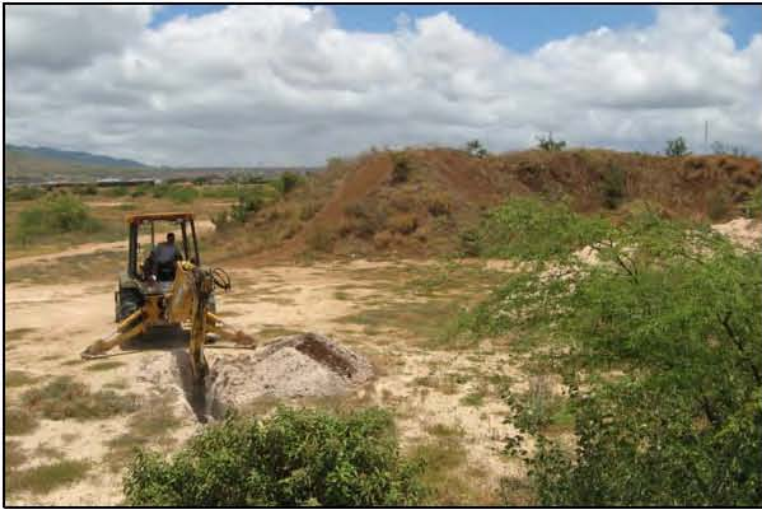
Figure 19. Stockpile 2, west side, backhoe for scale (note ORV jumps, view to north).
