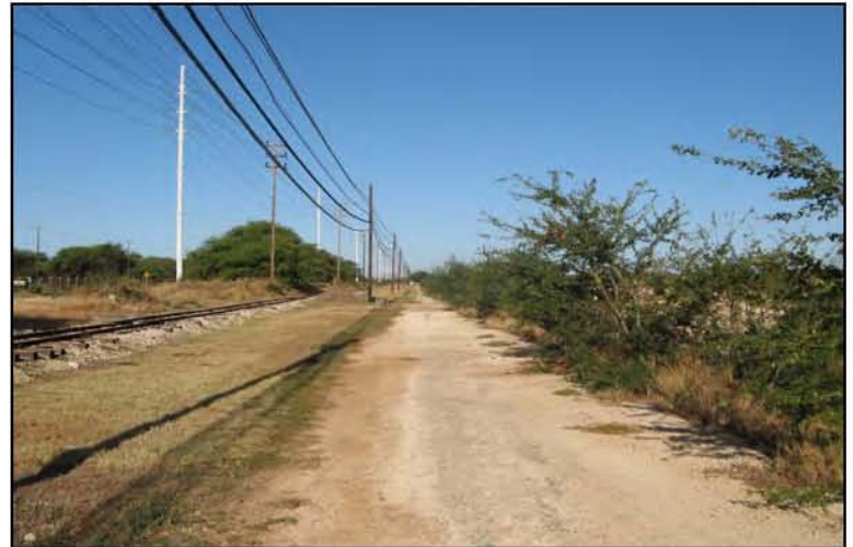
Figure 21. Access road between OR&L tracks and Borrow Pit (view to west).
