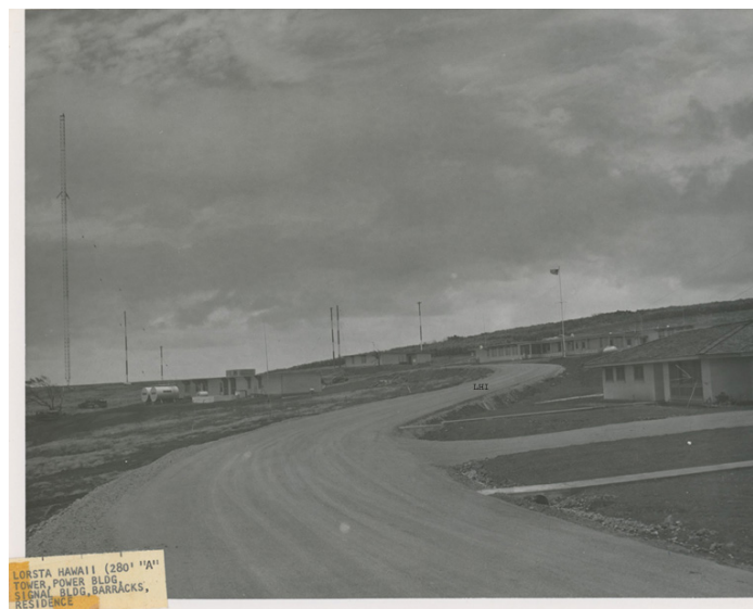
Photo of Newly Graded Road
