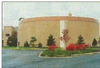
One of the digester tanks used to treat solids to make biosolids
