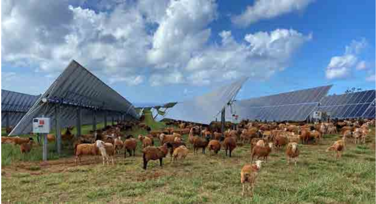
Photograph of typical sheep grazing operation within solar facility ( Lawai Solar + Storage )
