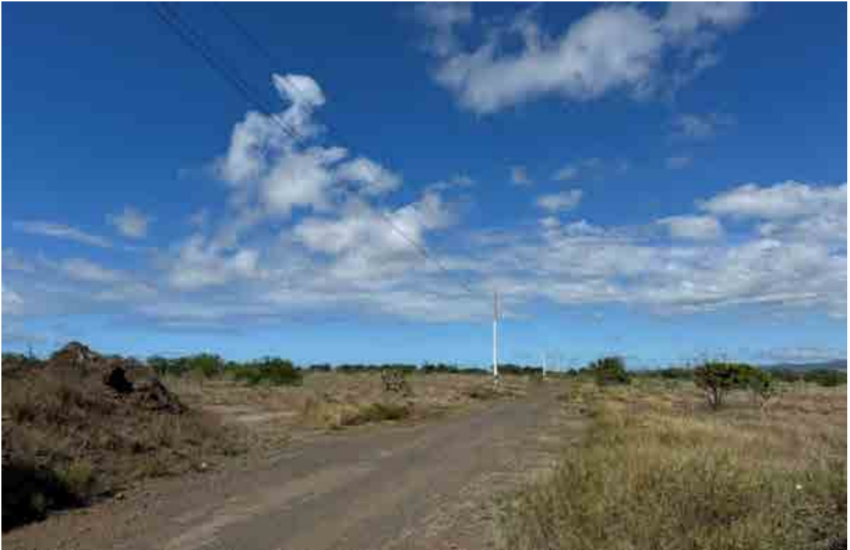
Photograph 10. Looking northeast along privately owned plantation road (9 th Street) and Maui Electric transmission line (September 6, 2024)
