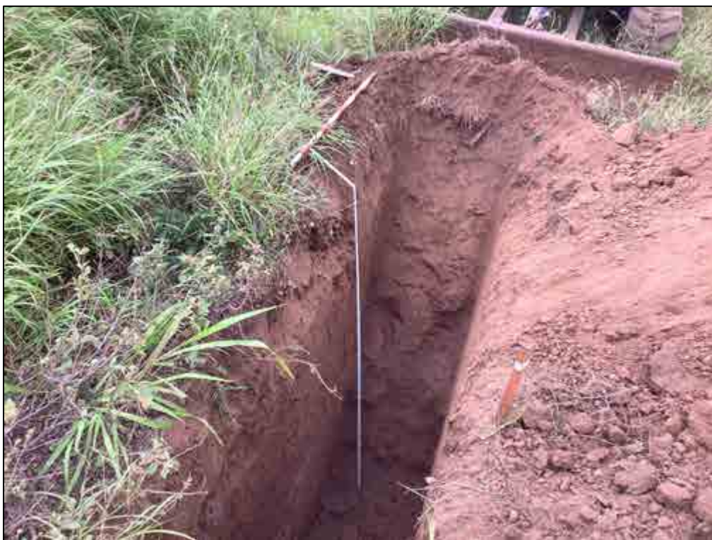
Figure 150. TP-8 observed stratigraphy (0.0-2.4 m), view to east
