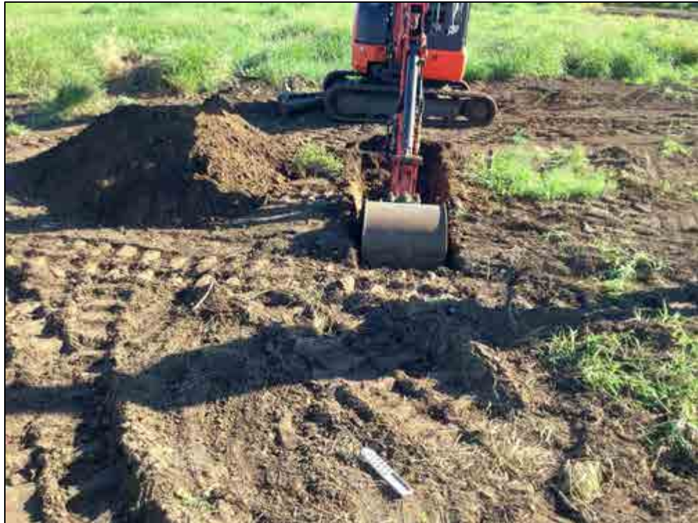
Figure 143. TP-1, overview of excavation, view to northeast
