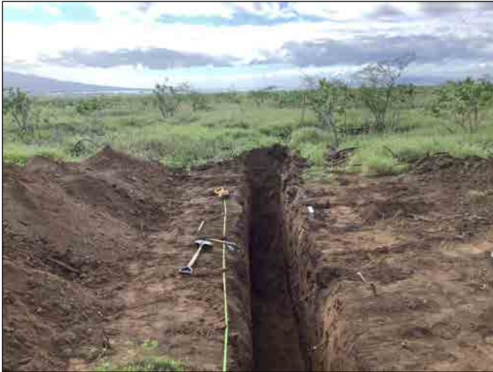
Figure 131. TE-31, overview of the general location, view to south
