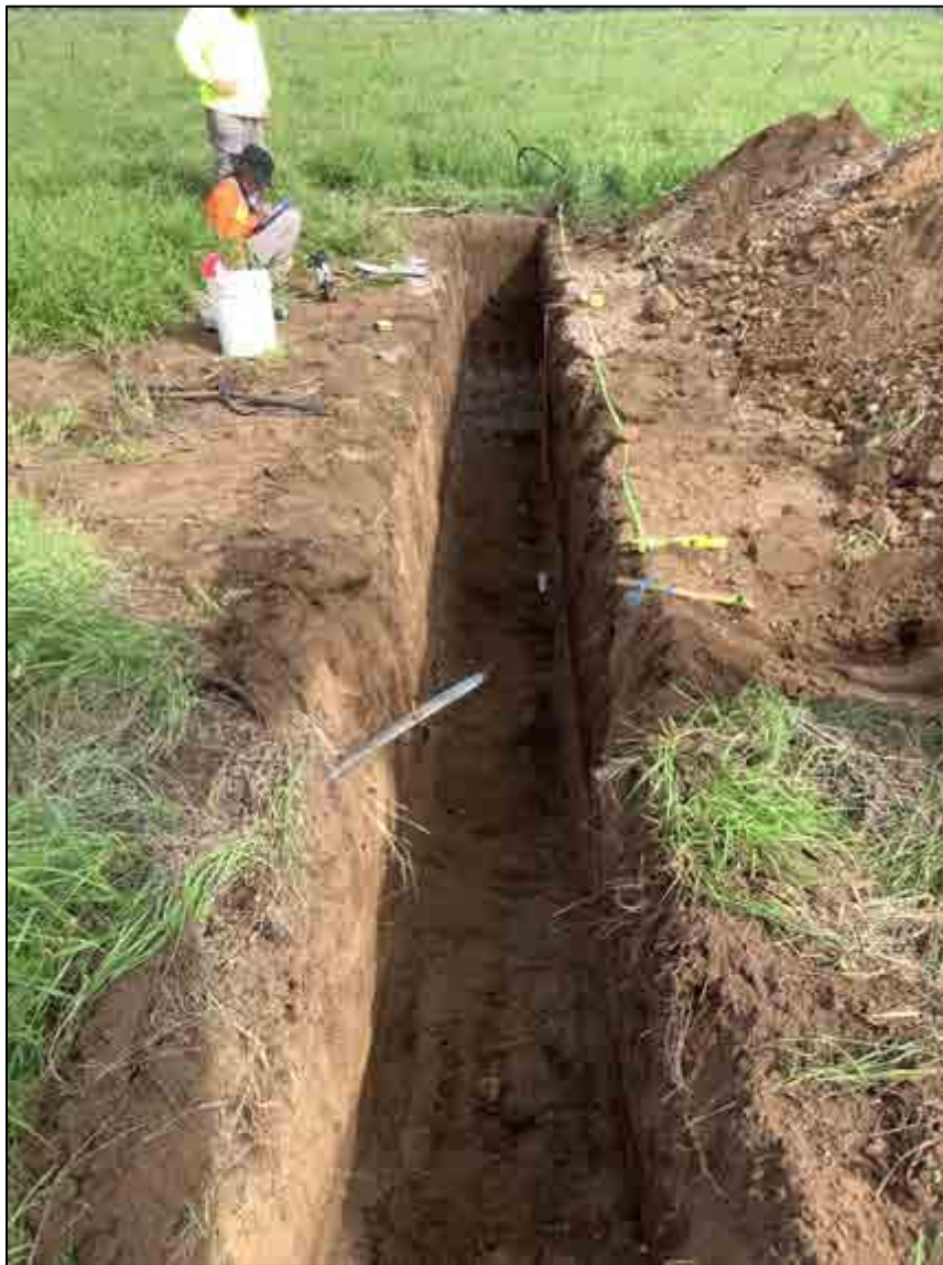
Figure 72. TE-17, overview of excavation area, view to north
