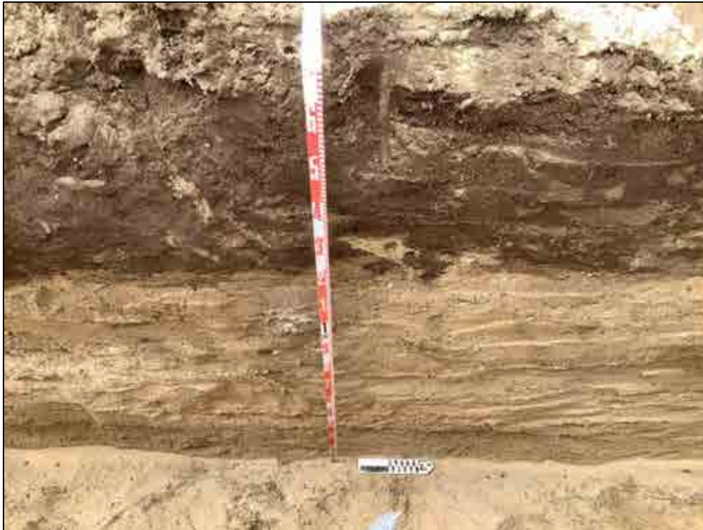
Figure 100. TE-23, close-up of the west wall
