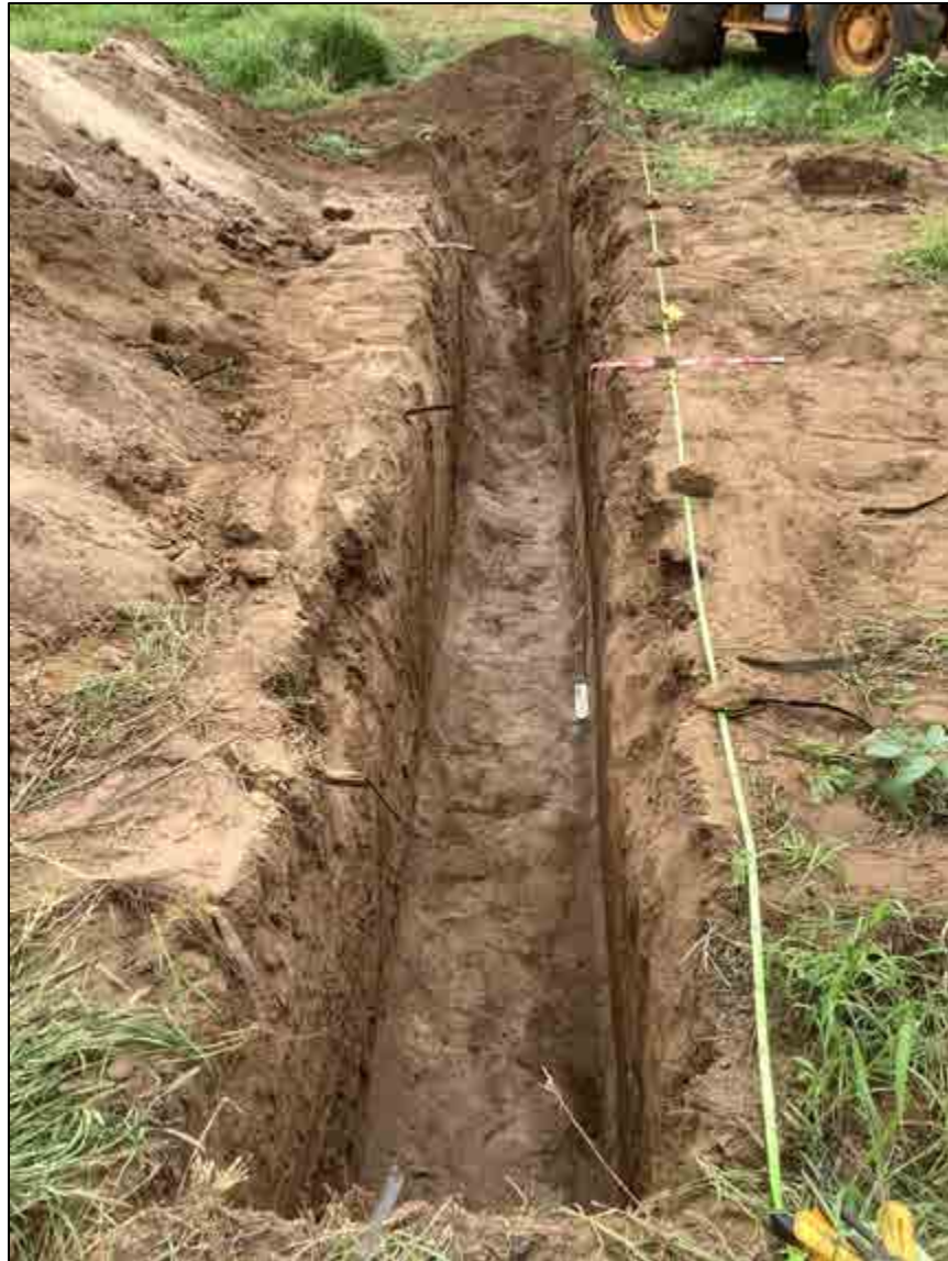
Figure 103. TE-24, overview of excavation area, view to south
