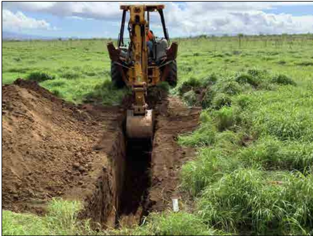
Figure 37. TE-9, overview of the general location, view to south
