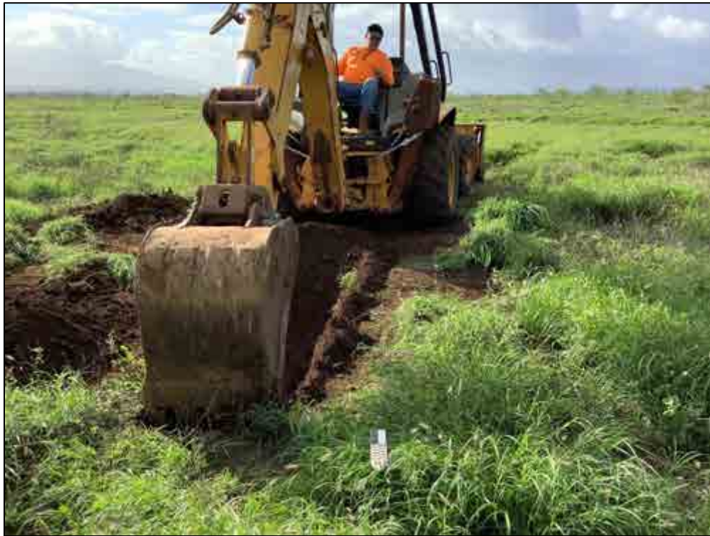
Figure 21. TE-5, overview of the general location, view to south
