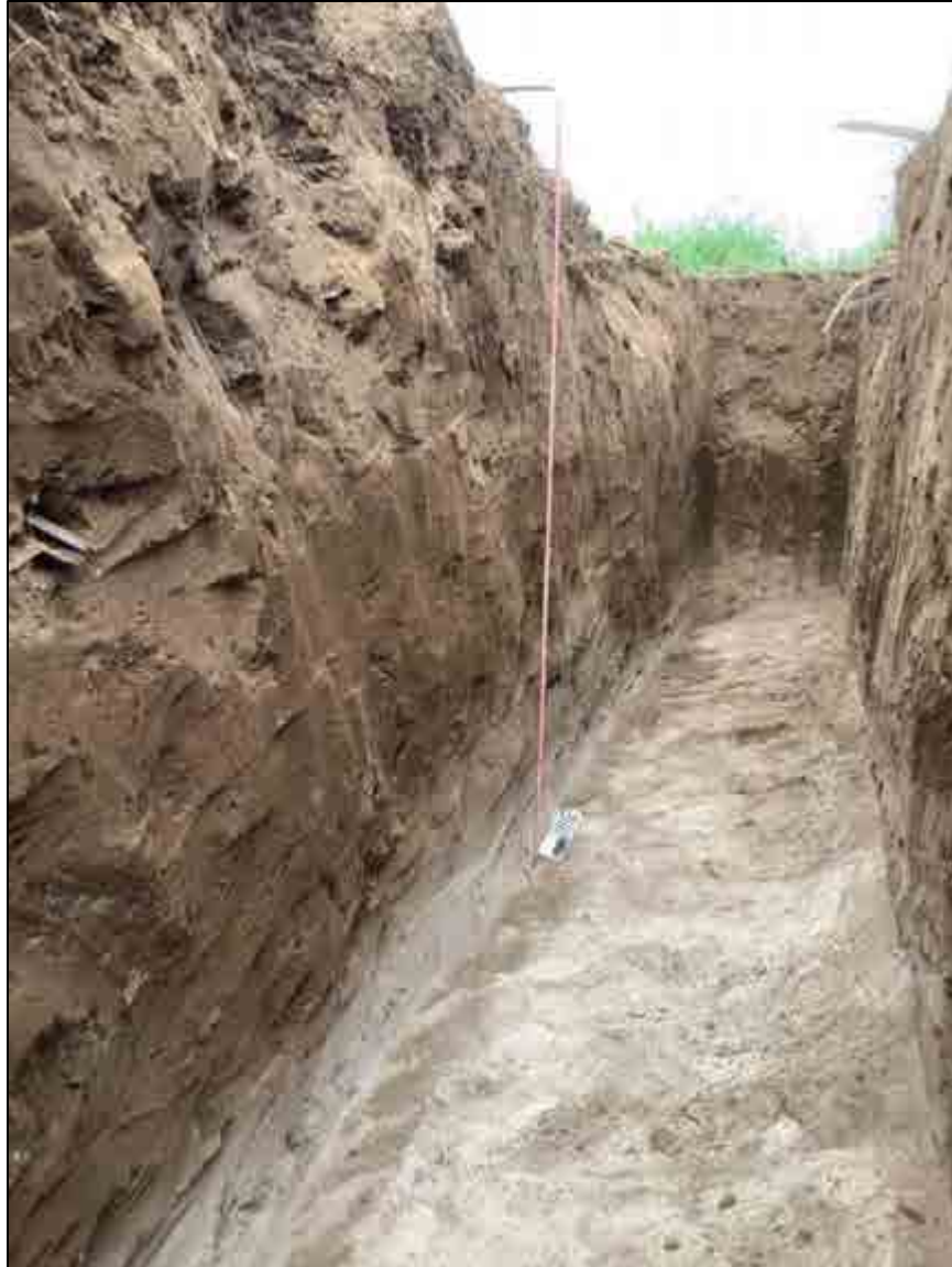
Figure 104. TE-24, oblique view of the west wall, view to northwest
