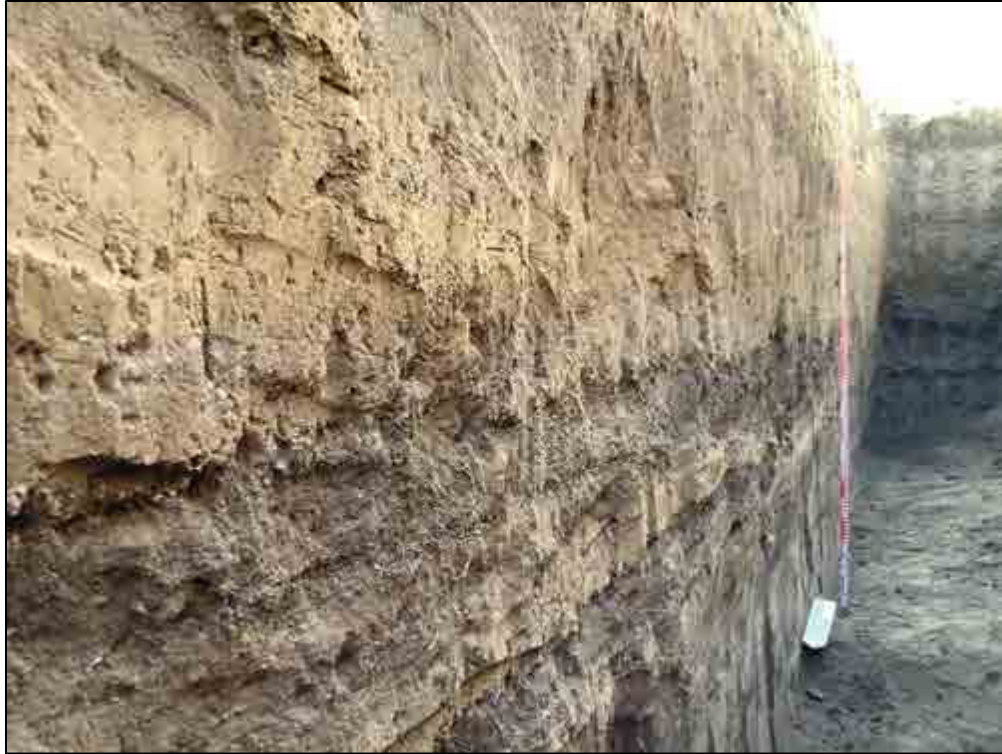
Figure 380. TE-92, oblique view of the east wall, view to southeast
