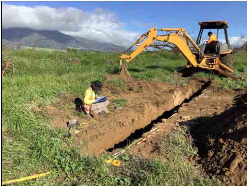
Figure 195. TE-47, overview of the general location, view to northwest
