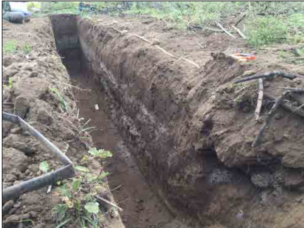
Figure 259. TE-62, overview of the east wall, view to southwest
