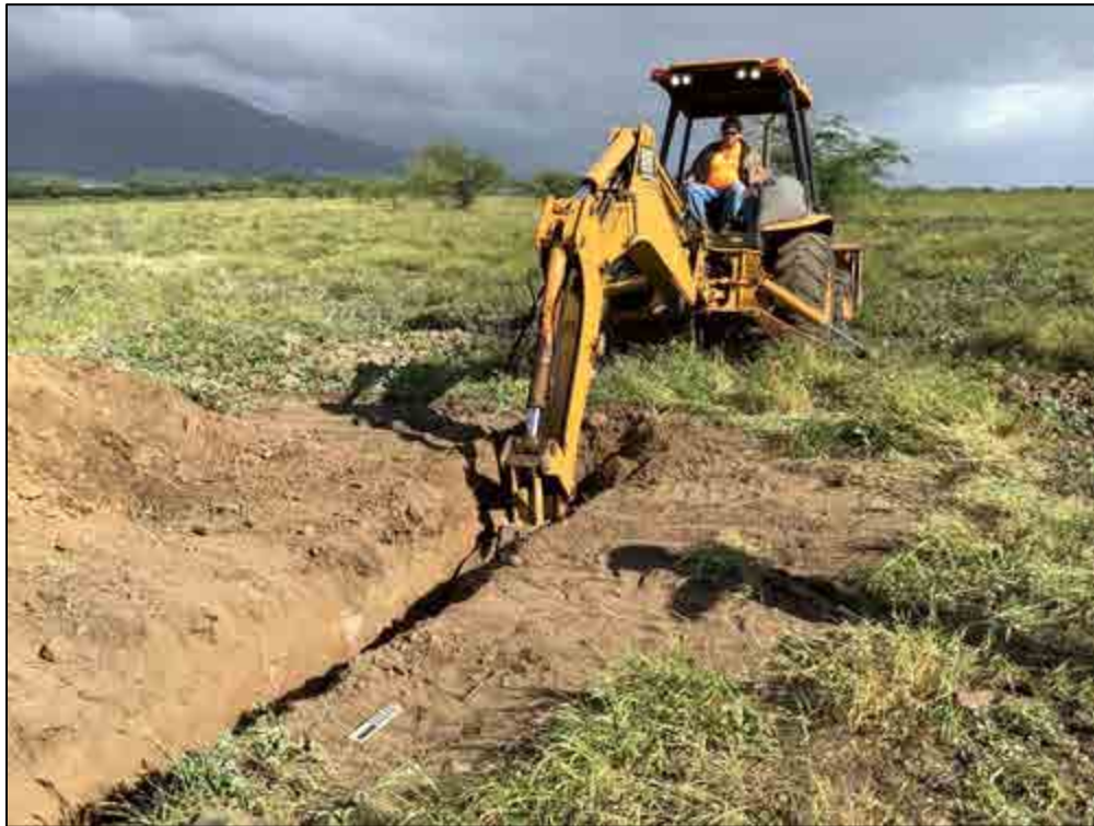
Figure 284. TE-69, overview of the general location, view to northwest
