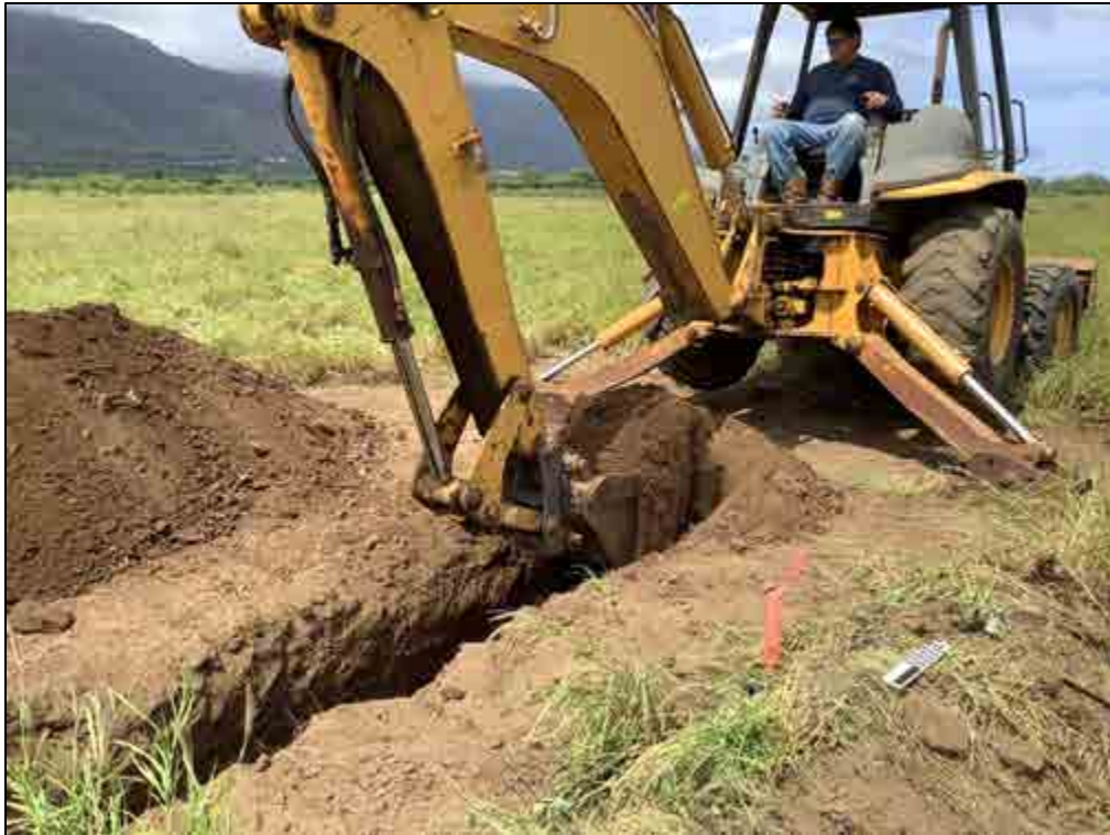
Figure 321. TE-78, overview of the general location, view to northwest
