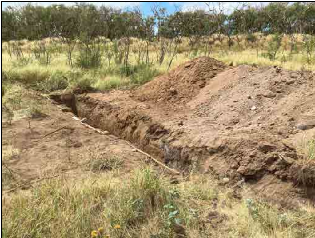
Figure 167. TE-142, overview of the general location, view to southwest
