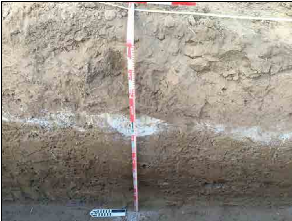
Figure 25. TE-106, close-up of the east wall, view to east
