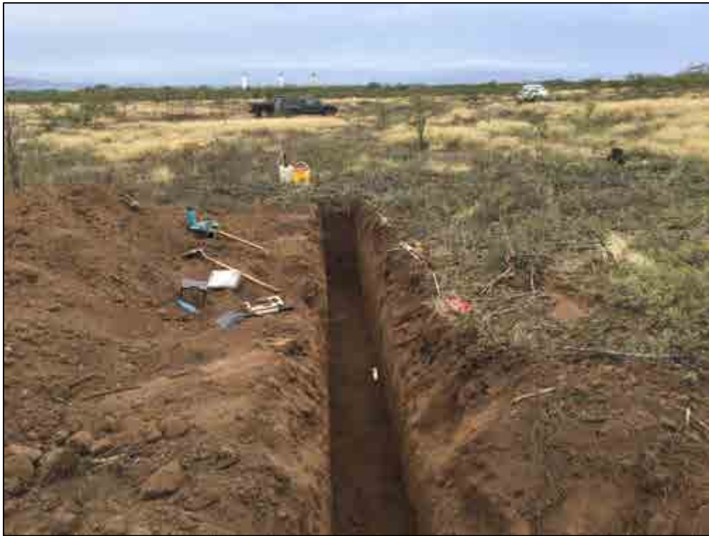
Figure 213. TE-153, overview of the general area, view to south
