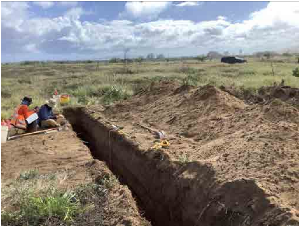
Figure 83. TE-121, overview of the general location, view to southwest
