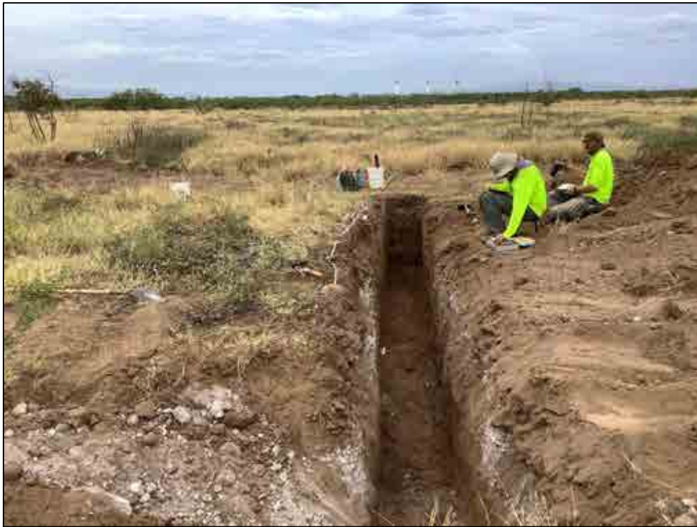
Figure 221. TE-155, overview of the general location, view to south
