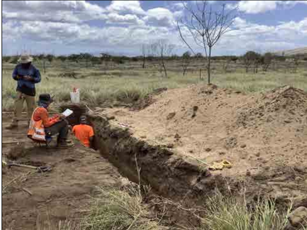
Figure 87. TE-122, overview of the general location, view to southwest
