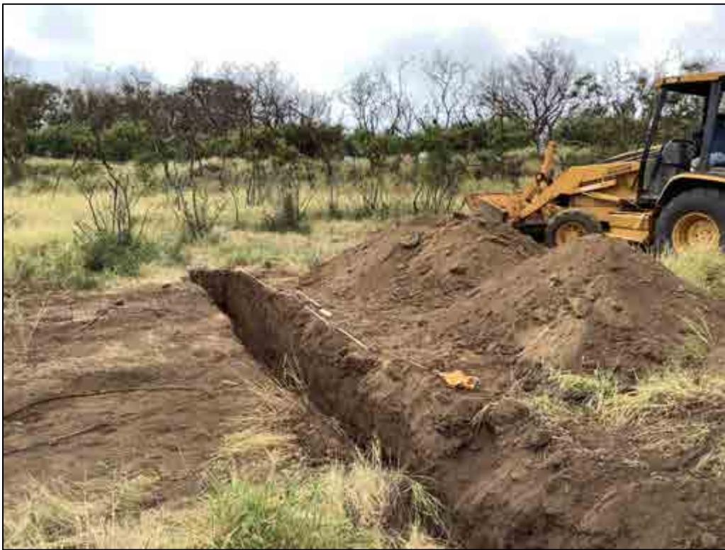
Figure 225. TE-156, overview of the general location, view to southwest
