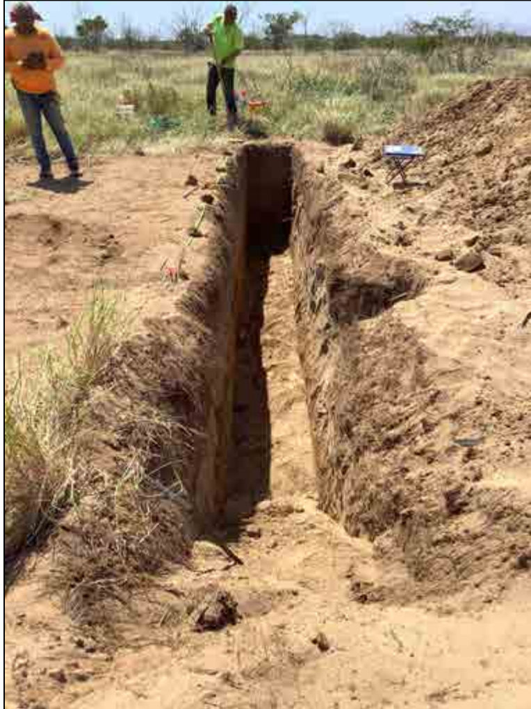
Figure 43. TE-111, overview of excavation area, view to south
