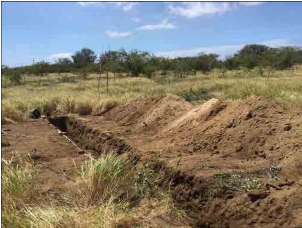
Figure 233. TE-158, overview of the general location, view to southwest
