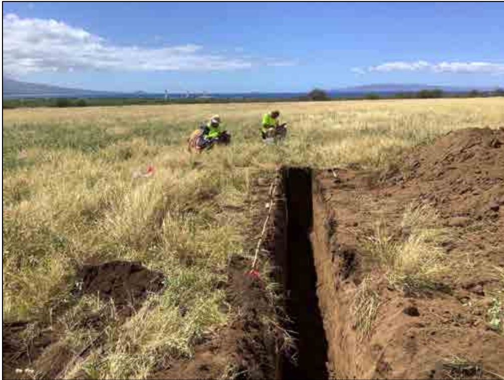
Figure 3. TE-101, overview of the general location, view to south
