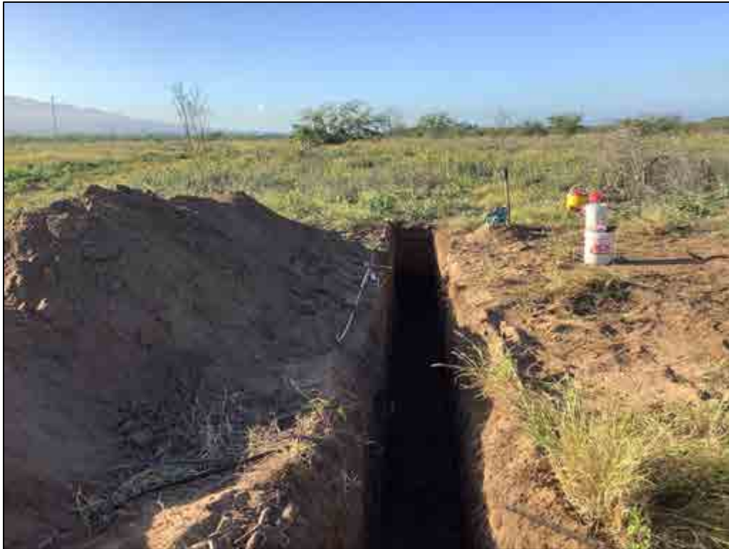
Figure 187. TE-147, overview of the general location, view to south
