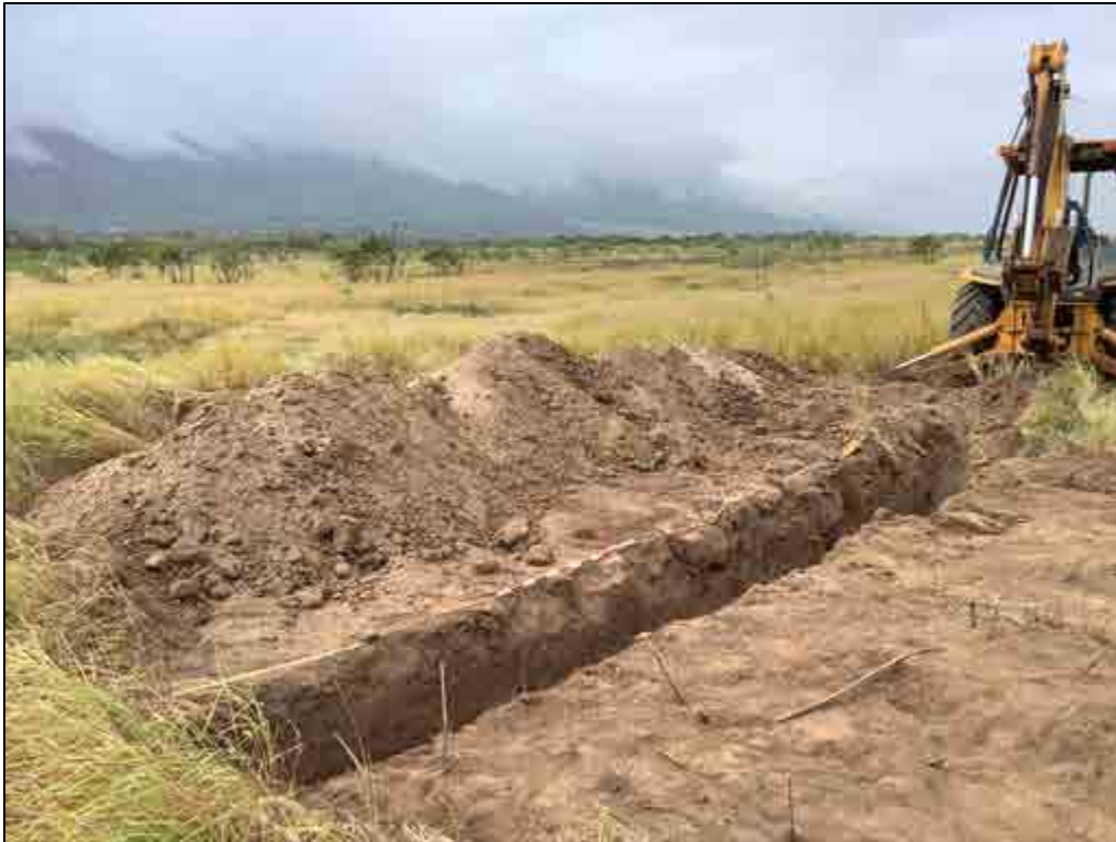
Figure 229. TE-157, overview of the general location, view to northwest
