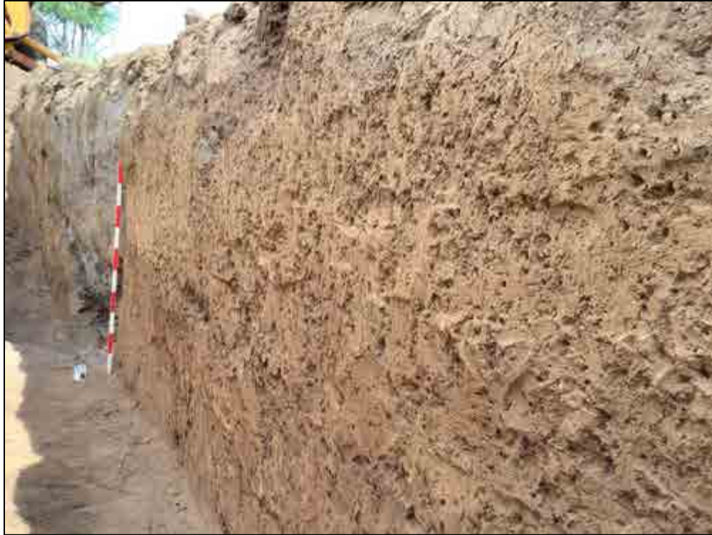
Figure 168. TE-142, oblique view of the east wall, view to northeast
