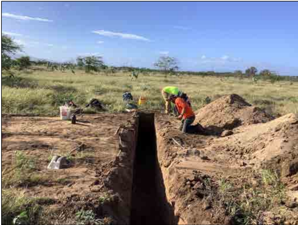
Figure 131. TE-133, overview of the general location, view to south
