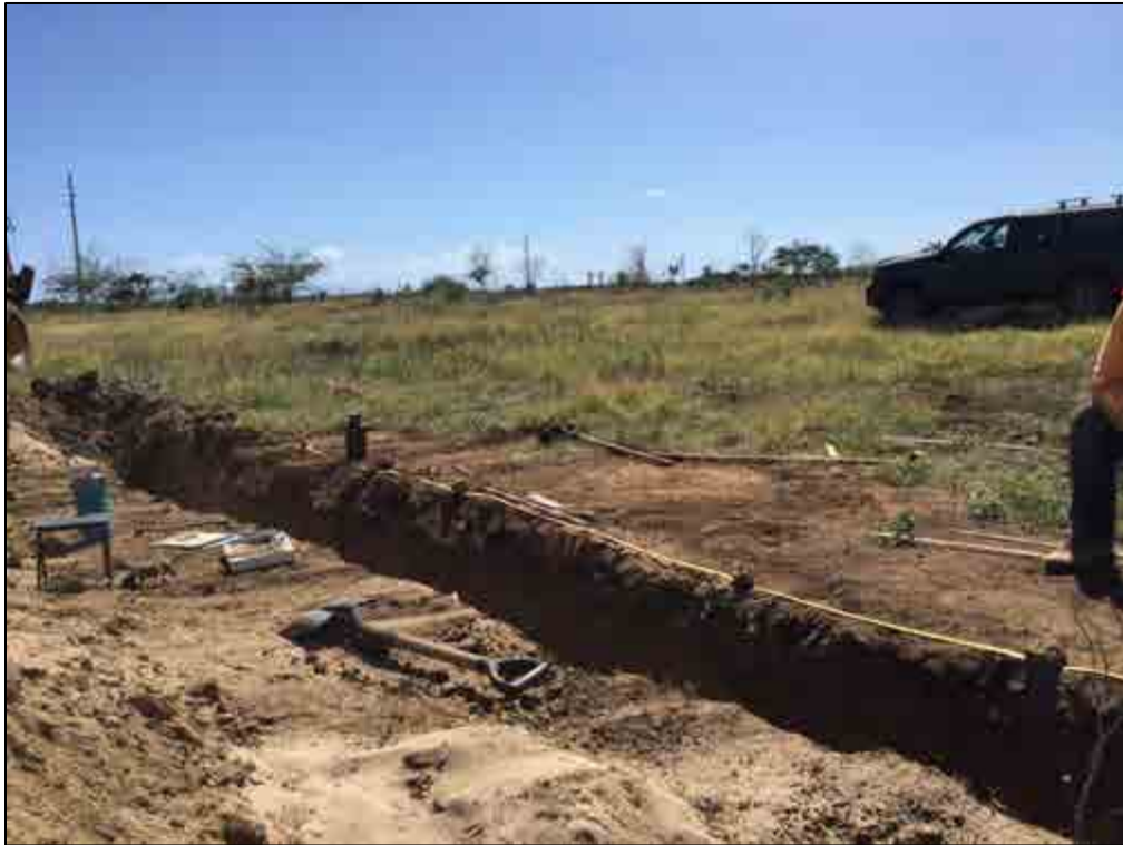
Figure 245. TE-161, overview of the general location, view to southwest
