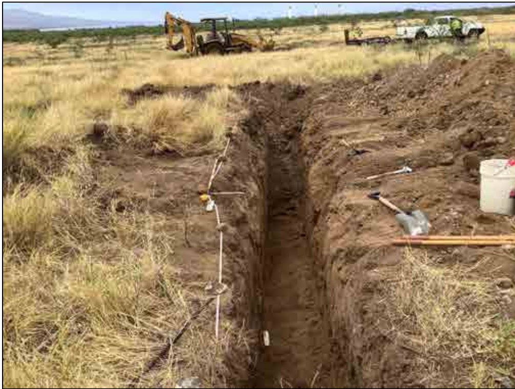
Figure 217. TE-154, overview of the general location, view to south
