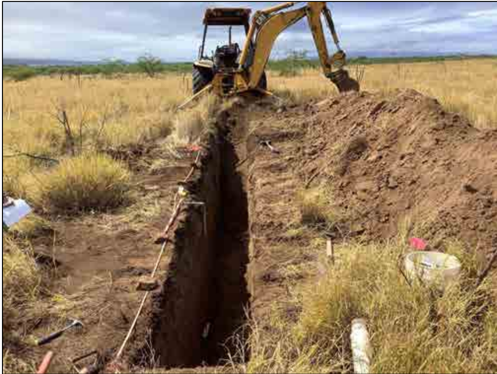
Figure 163. TE-141, overview of the general location, view to south
