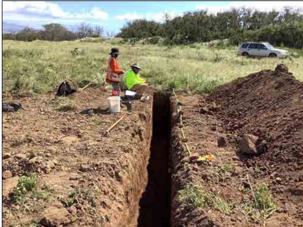
Figure 11. TE-103, overview of the general location, view to south
