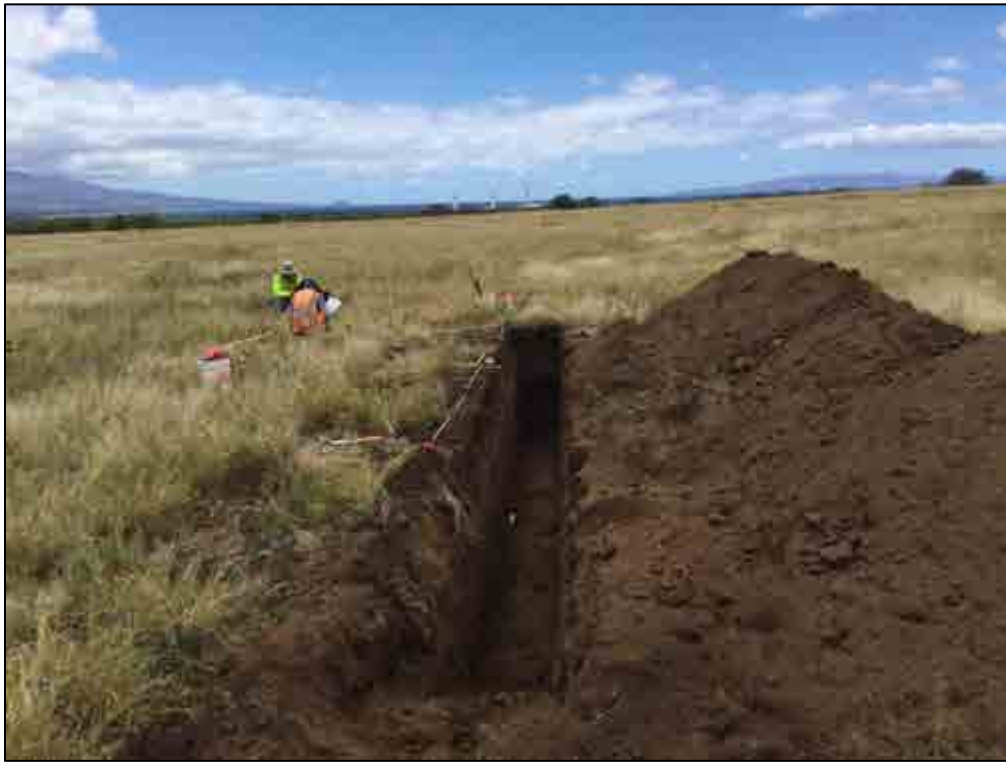
Figure 7. TE-102, overview of the general location, view to south
