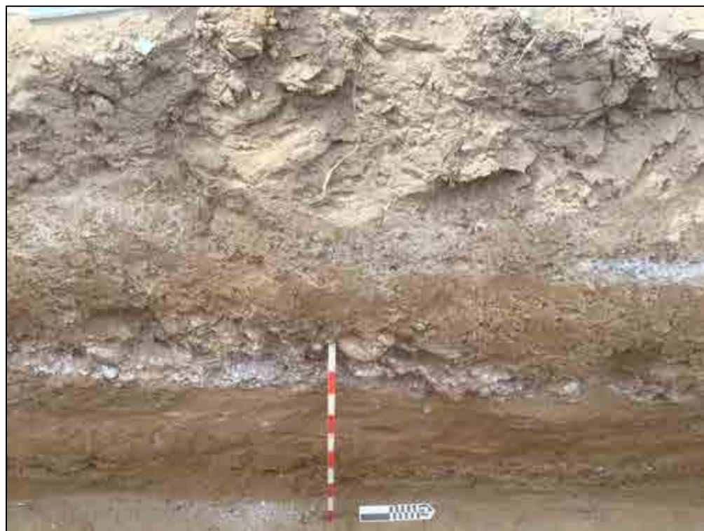
Figure 69. TE-117, close-up of the west wall, view to west
