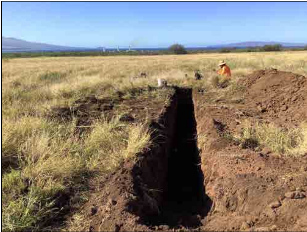
Figure 47. TE-112, overview of the general location, view to south
