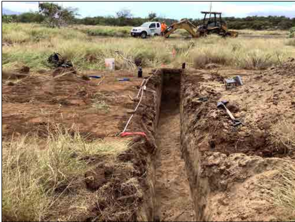
Figure 395. TE-198, overview of the general area, view to south
