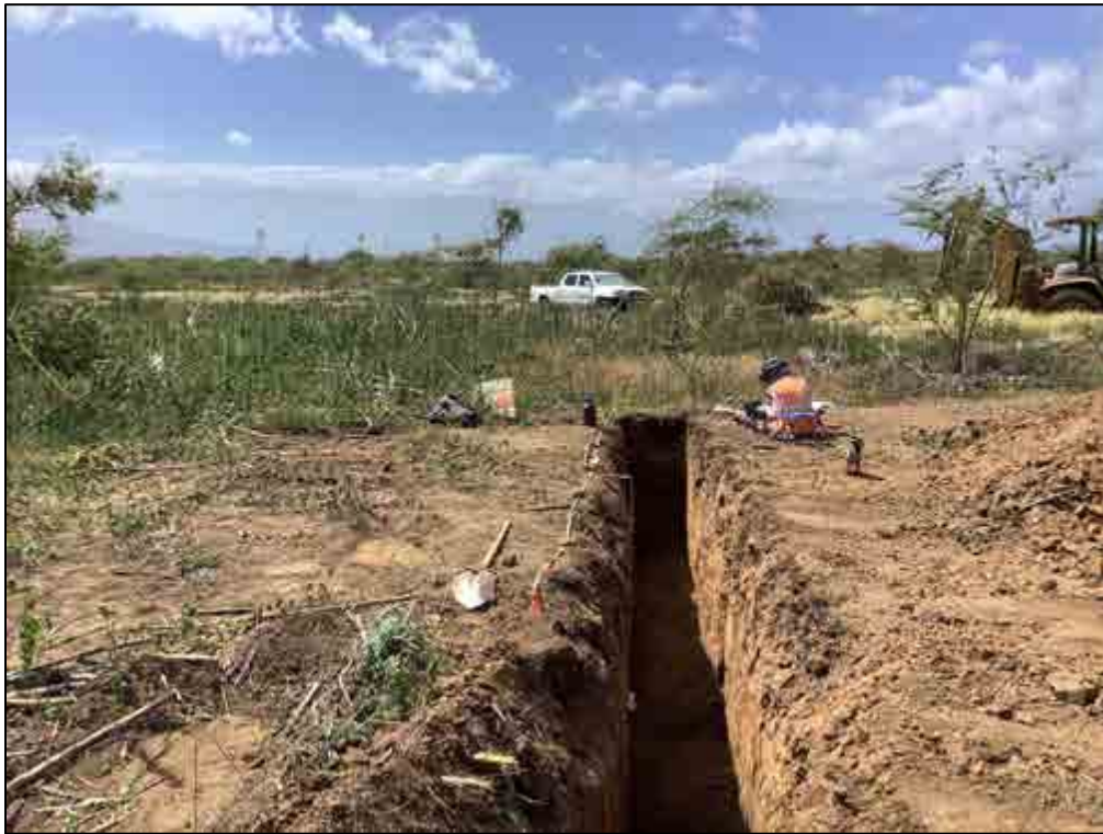
Figure 403. TE-200, overview of the general area, view to south
