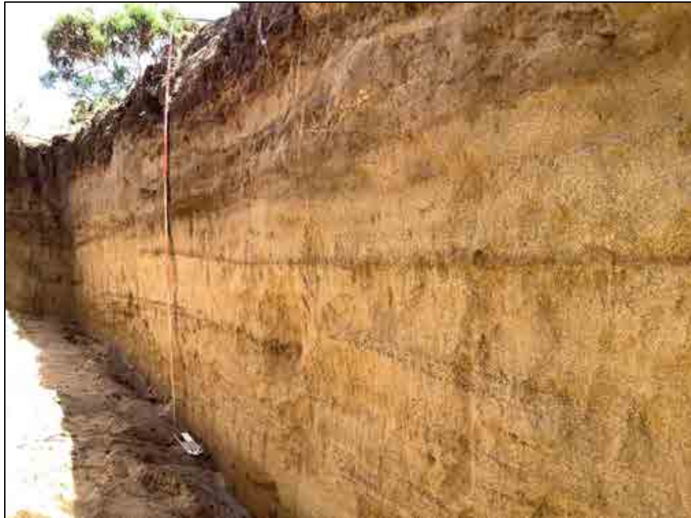
Figure 464. TE-215, oblique view of the west wall, view to southwest
