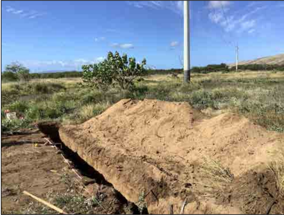
Figure 351. TE-187, overview of the general location, view to southwest
