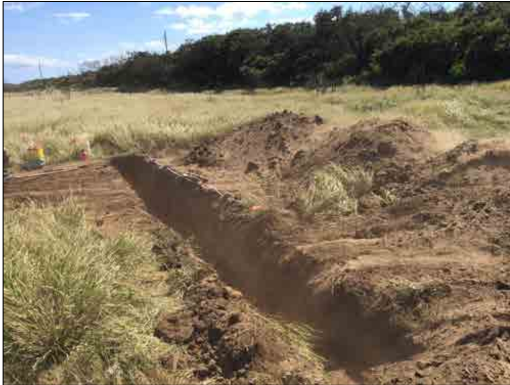
Figure 343. TE-185, overview of the general location, view to southwest
