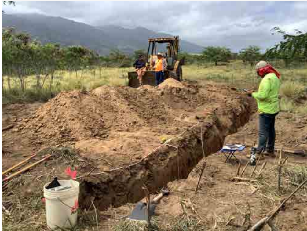
Figure 491. TE-222, overview of the general location, view to northwest
