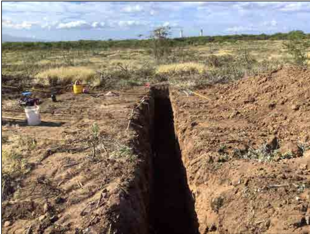
Figure 415. TE-203, overview of the general area, view to south
