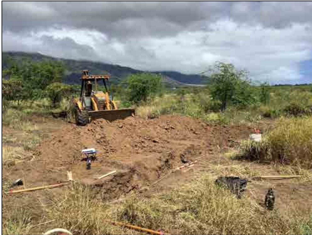
Figure 499. TE-224, overview of the general location, view to northwest
