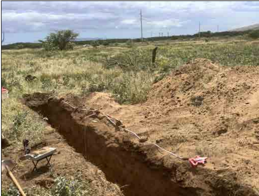
Figure 299. TE-174, overview of the general location, view to northwest
