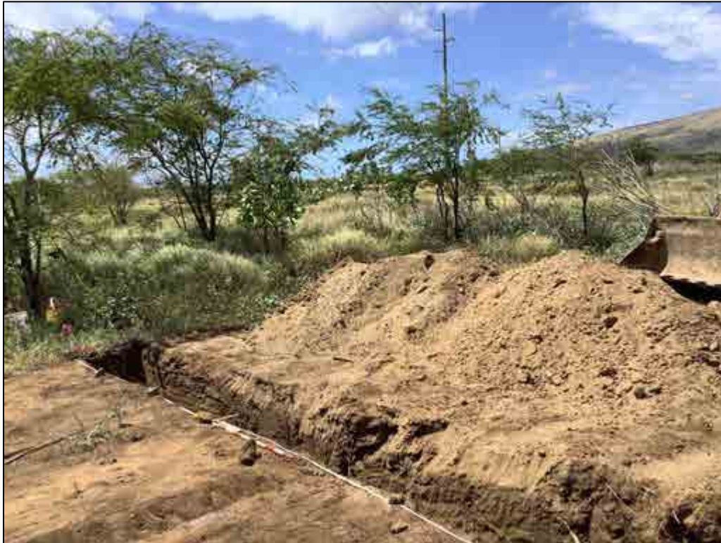
Figure 303. TE-175, overview of the general location, view to southwest
