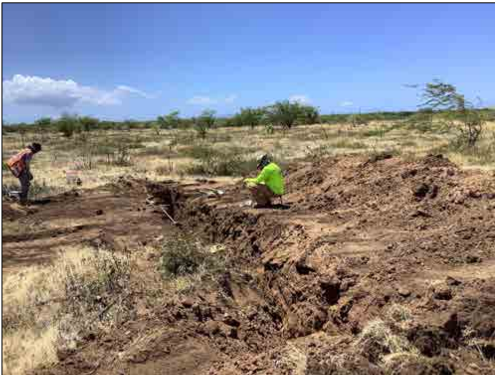
Figure 335. TE-183, overview of the general location, view to southwest
