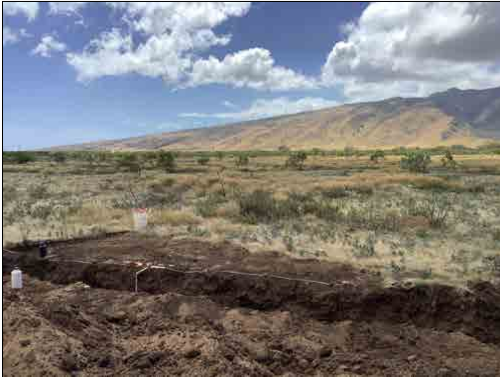
Figure 379. TE-194, overview of the general location, view to southwest
