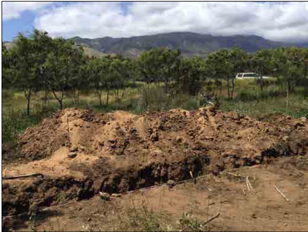
Figure 520. TE-229, overview of the general location, view to northwest
