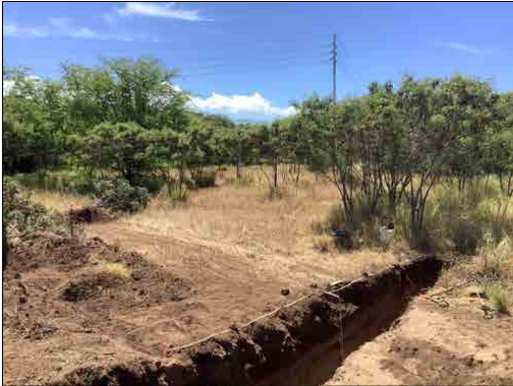
Figure 391. TE-197, overview of the general area, view to southeast
