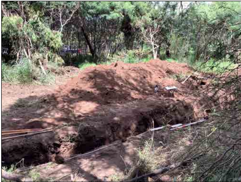
Figure 512. TE-227, overview of the general location, view to northwest
