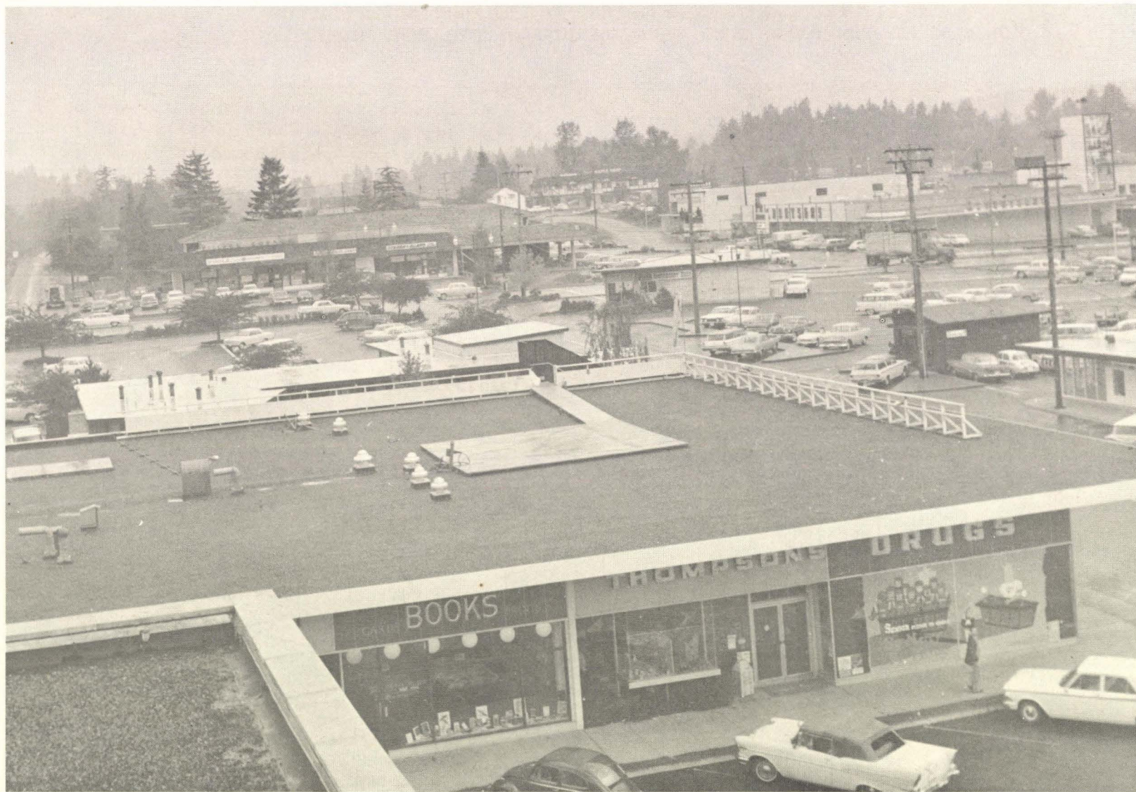
FIGURE 15. ROOFTOP HELIPORT, BELLEVUE, WASHINGTON, SHOWING 24' x 24' LOAD DISTRIBUTION PAD ON BUILT-UP ROOF AND HANDRAILS OR SAFETY BARRIERS
