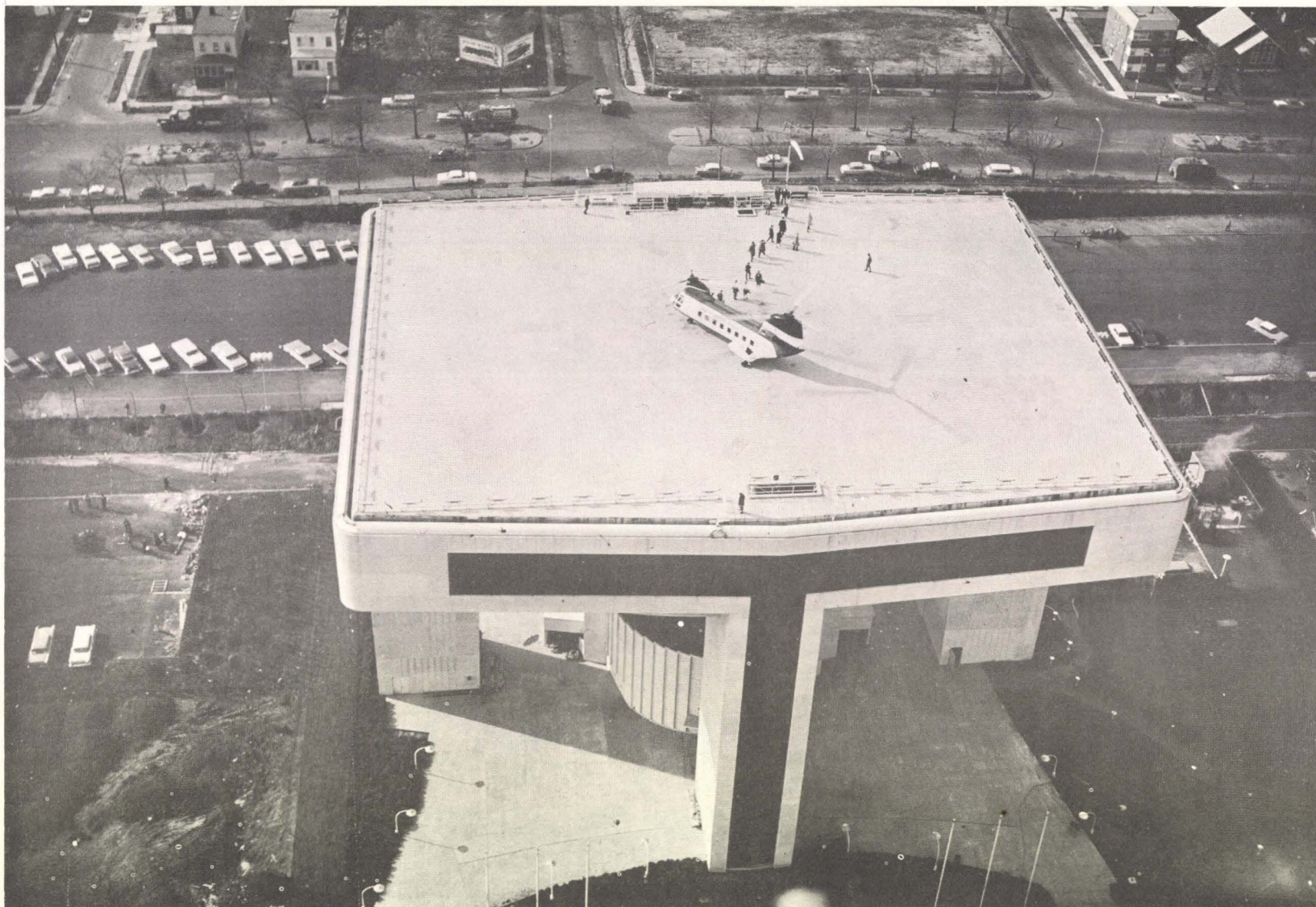
FIGURE 14. ROOFTOP HELIPORT, WORLD'S FAIR 1964, NEW YORK, NEW YORK. LANDING AND TAKEOFF AREA IS 200' x 150' AND IS 120' ABOVE THE GROUND.
